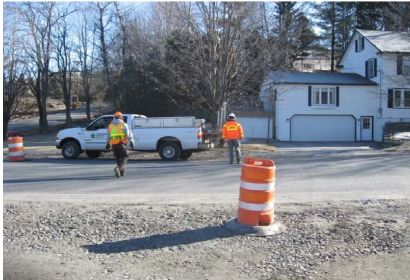
Location of SB-K/MW-4, facing east
