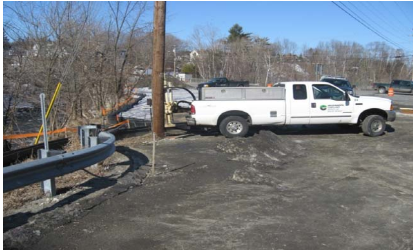
Installation of SB-B/MW-1, facing northwest
