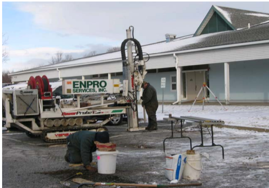
Drilling Monitoring Well MW08-4
