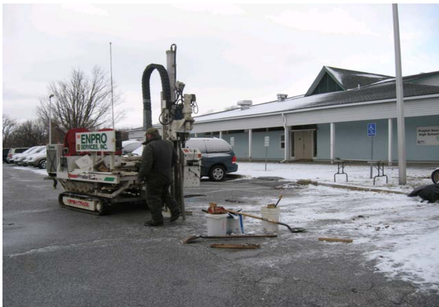
Drilling Monitoring Well MW08-3
