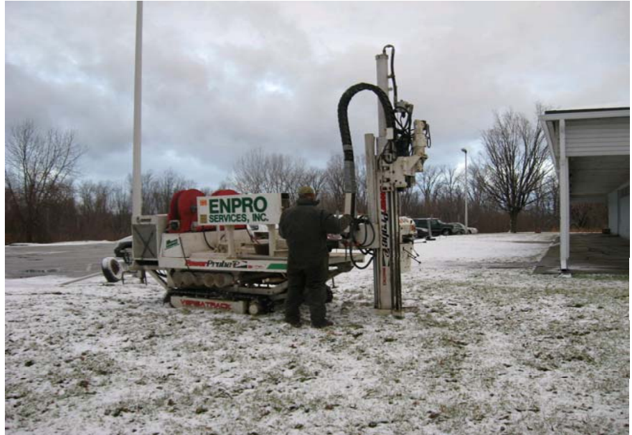
Drilling Monitoring Well MW08-2
