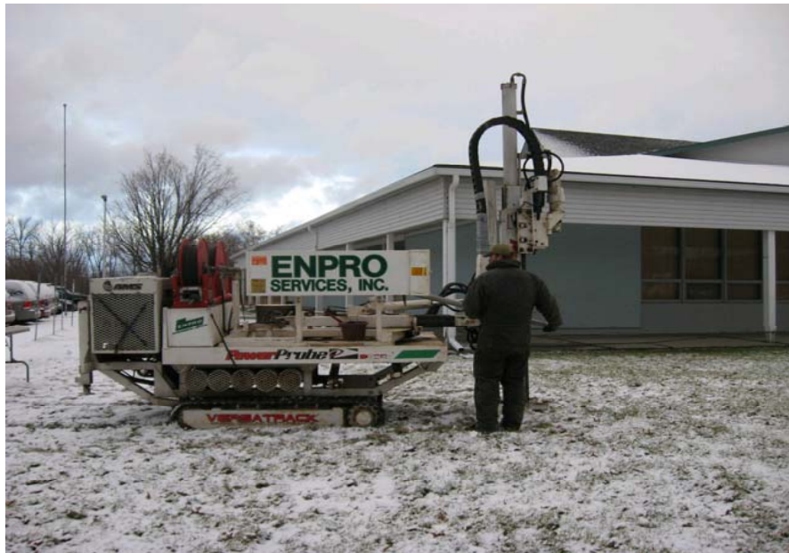
Drilling Monitoring Well MW08-1
