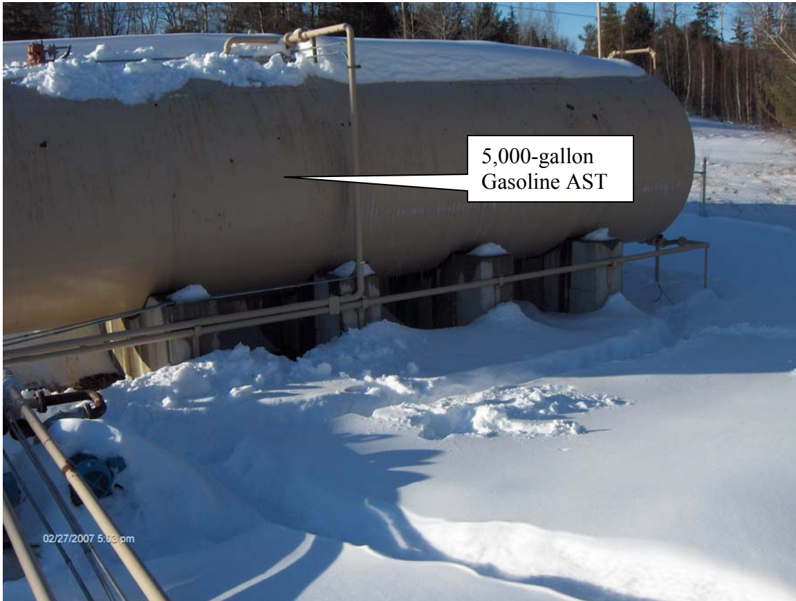
FP&H BULK STORAGE FACILITY – DERBY, VERMONT (Containment Berm covered with Gas contaminated snow – View toward North)
