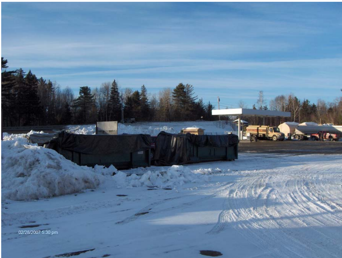
FP&H BULK STORAGE FACILITY – DERBY, VERMONT (Poly-lined dumpsters to contain contaminated snow – View Toward North)
