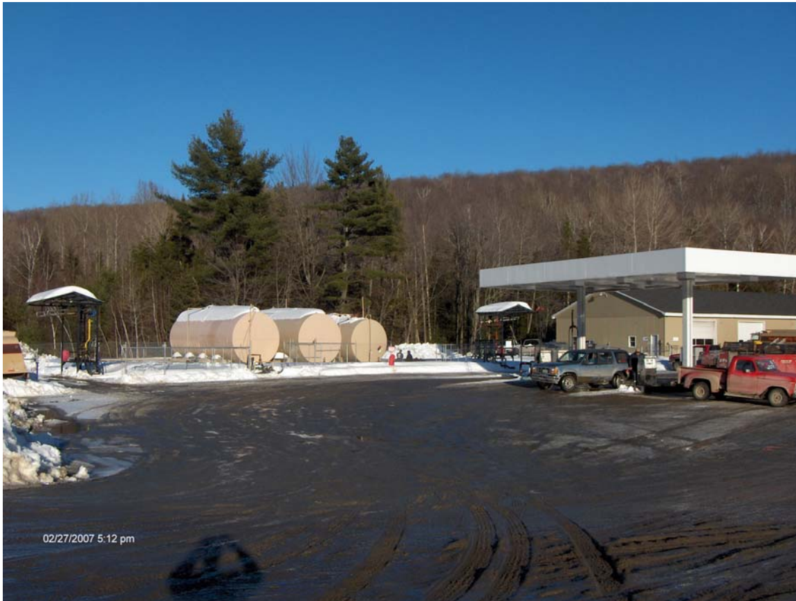
FP&H BULK STORAGE FACILITY – DERBY, VERMONT (Site Overview – View Toward North-Northeast)
