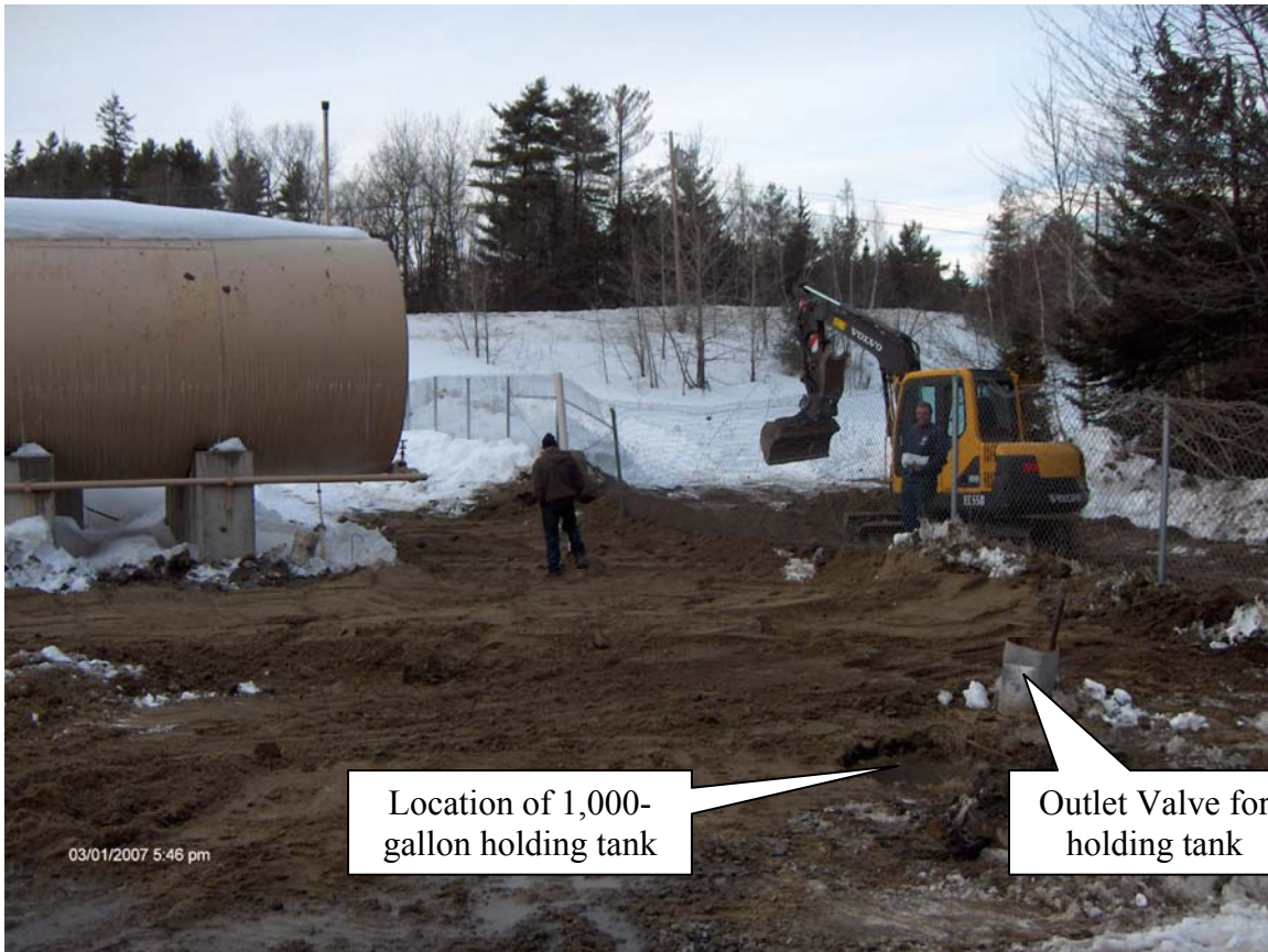
FP&H BULK STORAGE FACILITY – DERBY, VERMONT (Berm area up to grade with clean fill – View toward Northwest)
