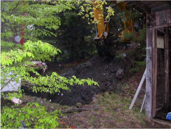
Start of soil excavation at base of slope.
