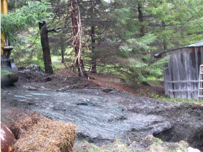
View looking north of ledge immediately below ground surface.
