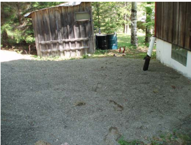
Backfilled excavation pit. Note standpipe installed in the event future remedial actions are warranted.
