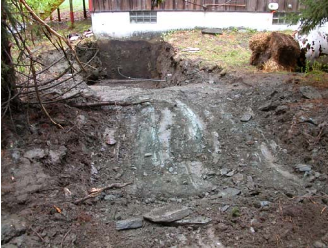
View looking west of excavation from pit at house.
