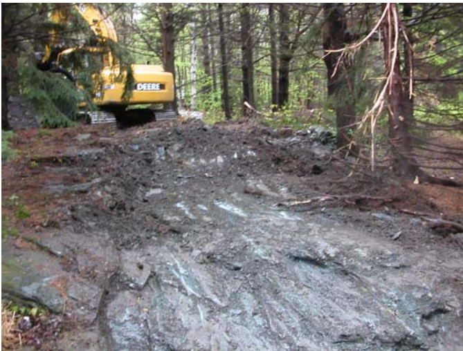
View looking west of excavation in vicinity of former AST location.
