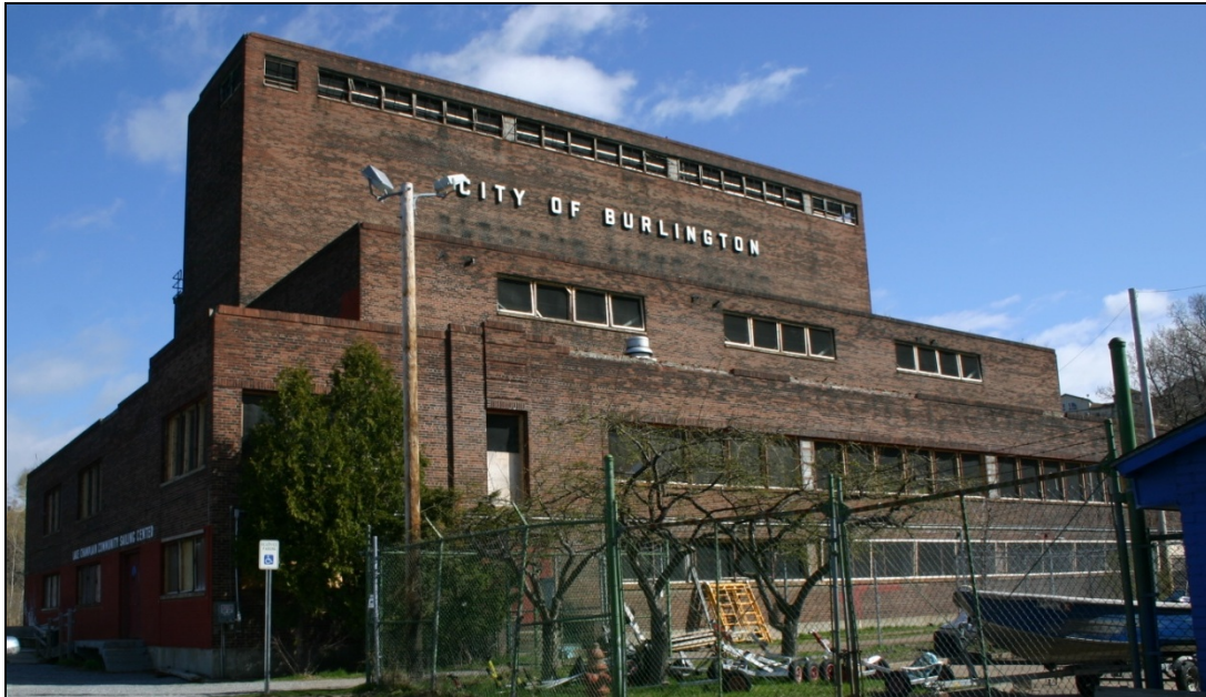
Moran Plant, S elevation (view NE)
