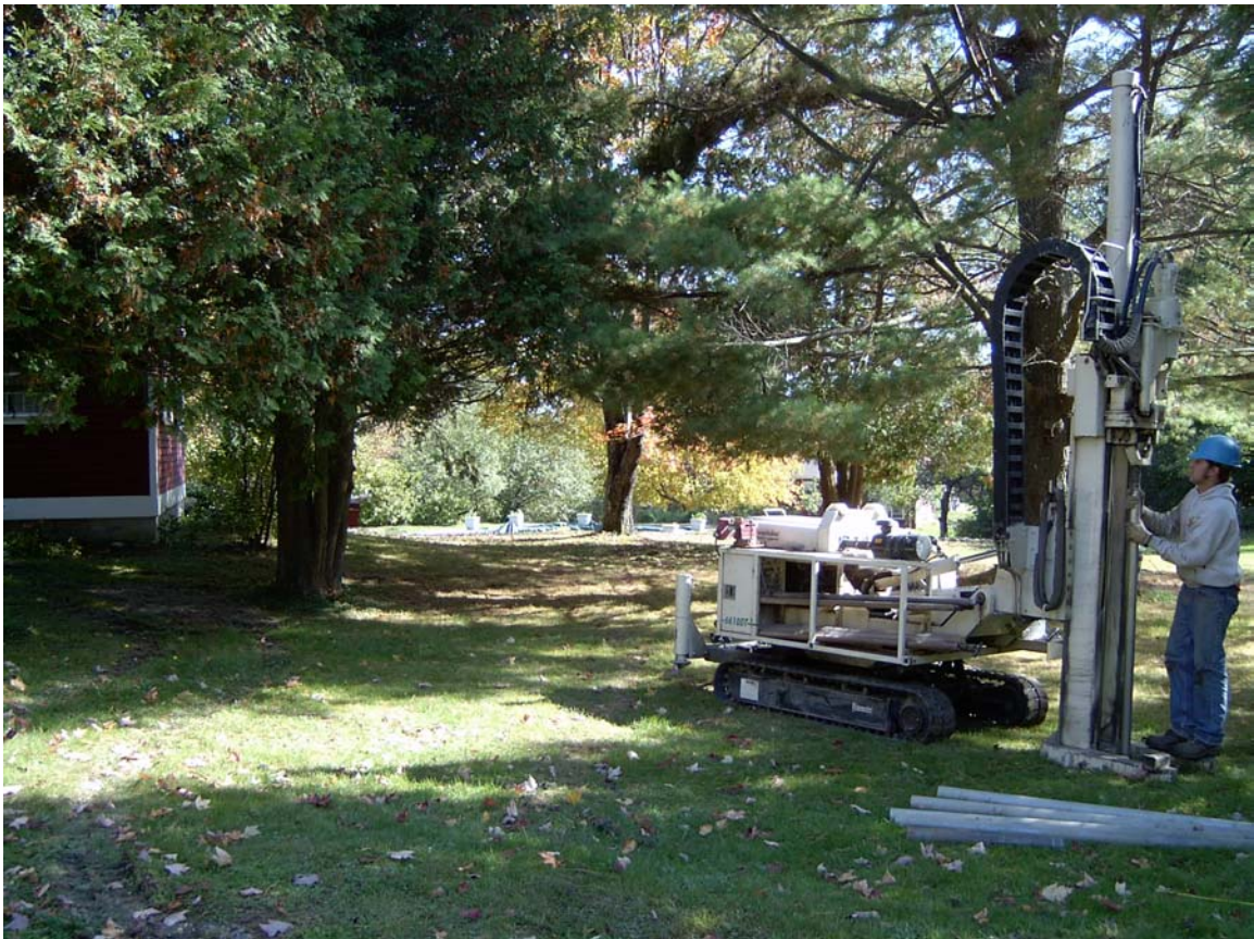
TEN ACRES LODGE – STOWE, VERMONT (Installation of MW-2 – View Toward North)
