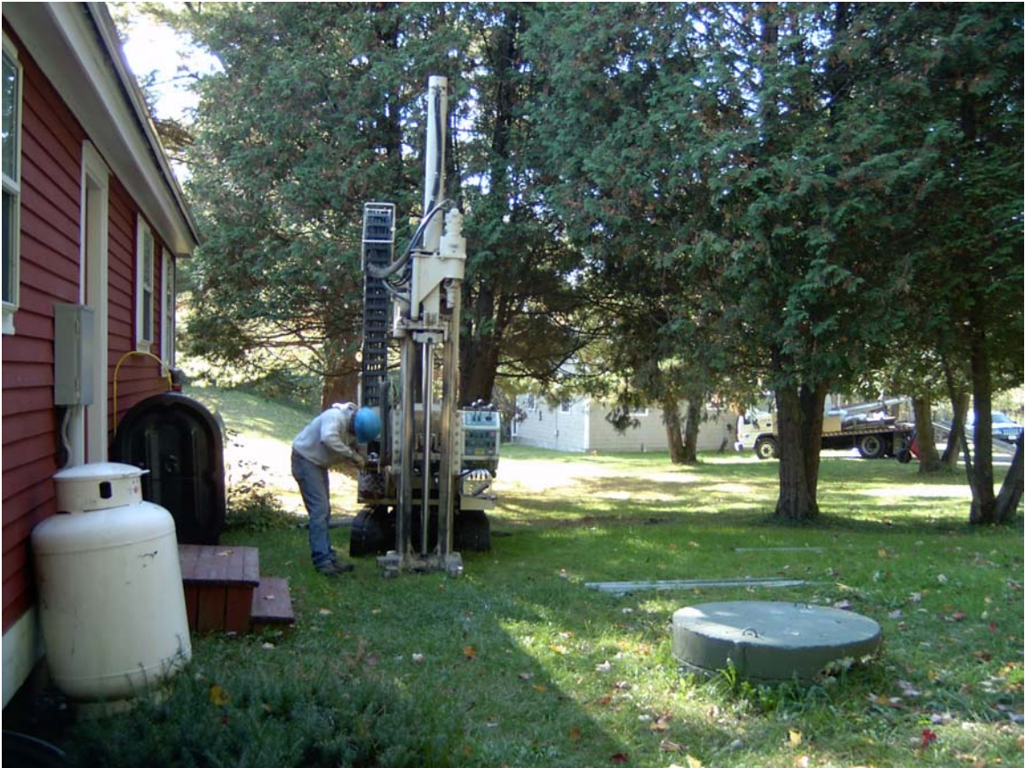
TEN ACRES LODGE – STOWE, VERMONT (Installation of MW-1 and Location of MW-2, and MW-3 – View Toward East)
