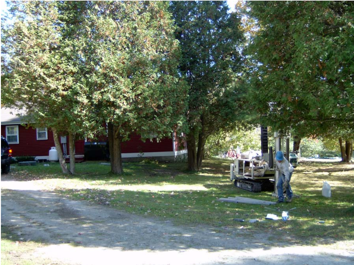
TEN ACRES LODGE – STOWE, VERMONT (Installation of MW-3 – View Toward North)
