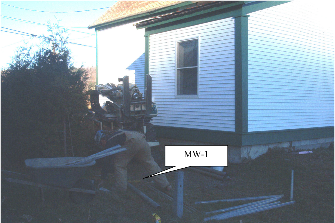
FERRY STREET (MW-1 Installation – View Toward North)
