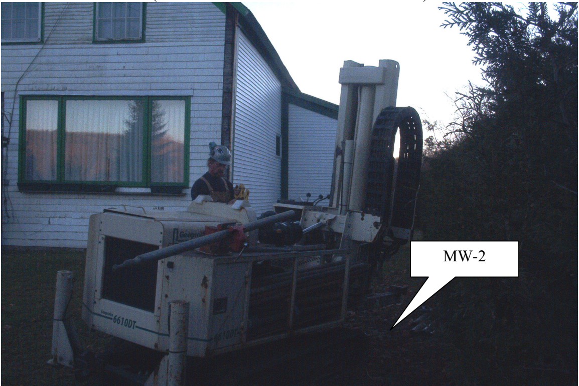
FERRY STREET (MW-2 Installation – View Toward South)
