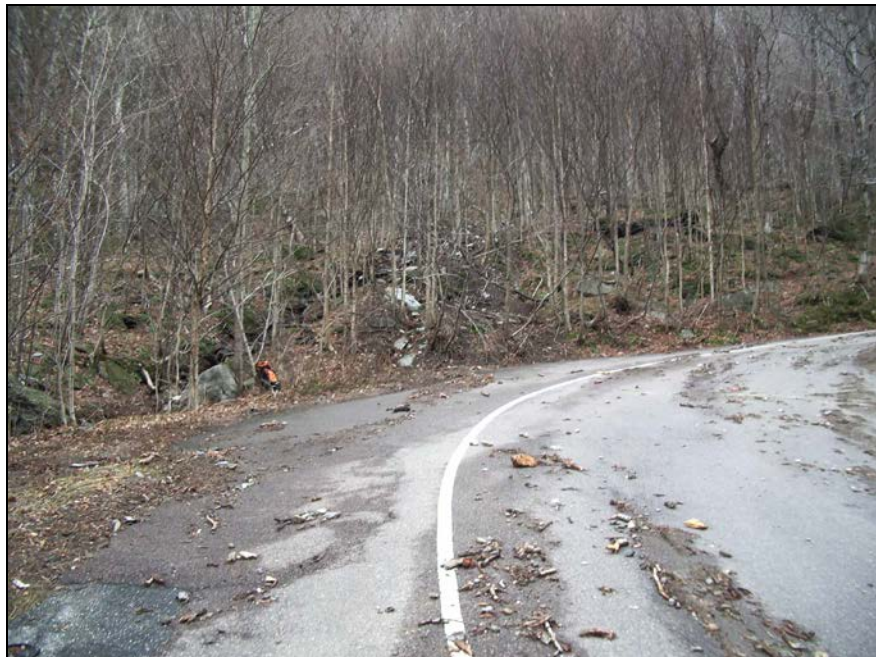
Figure 7.15. Debris flow that reached Vermont Rt. 108 at “S” turns. This slope failure occurred during a rain and snowmelt event of November 14 or 15, 2006. Snout of debris flow in center background.
