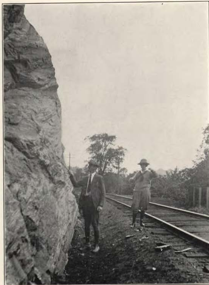
Chlorite schist overlying Barnard gneiss. R. R. cut two miles north of village, Bethel. Head of hammer at line of contact.
