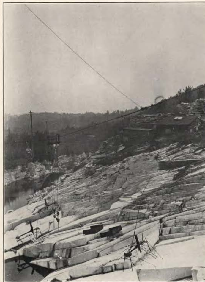
Granite quarry, Christian Hill, Bethel. Showing sheet structure and easterly dip.
