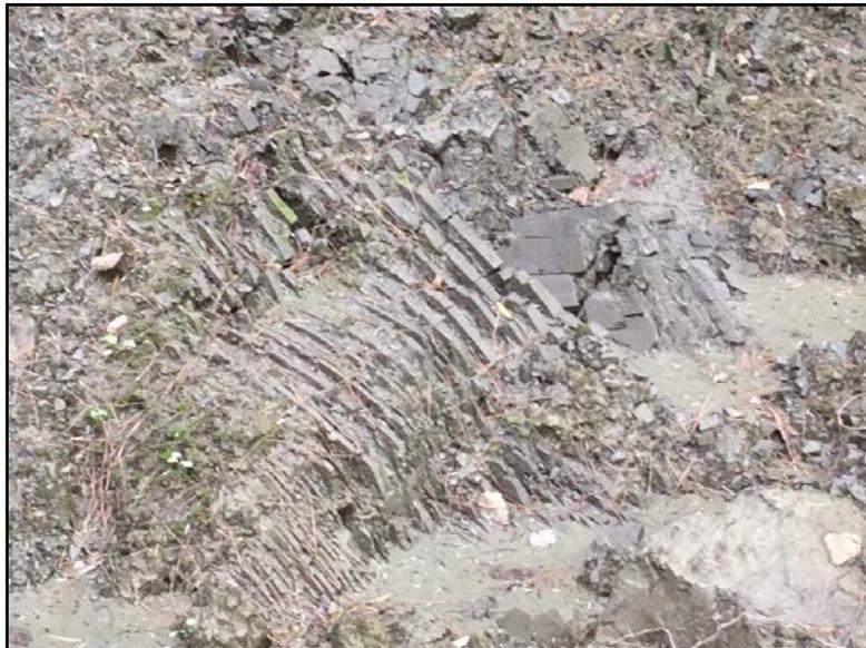
**Figure 14:** Slumped deposit of varved silt and clay adjacent to Barber Farm Road in Richmond. These cohesive sediments can be very strong when dry, but can weaken and slump when wet.
