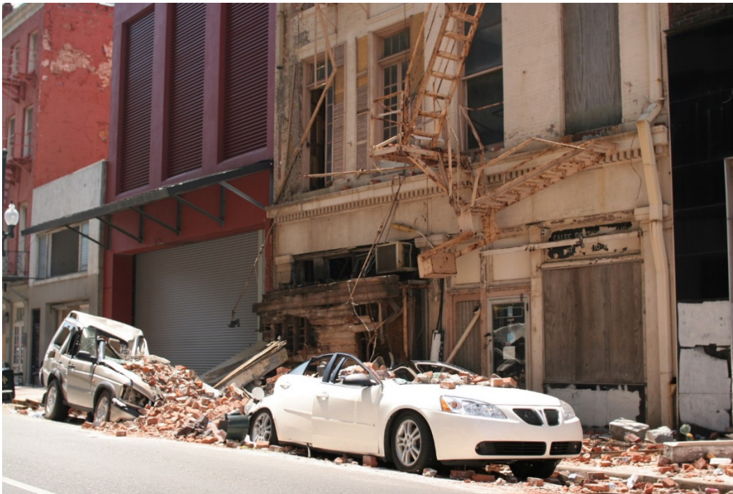
Figure 2. URM Building Damage New Orleans, LA Hurricane Katrina 2005
