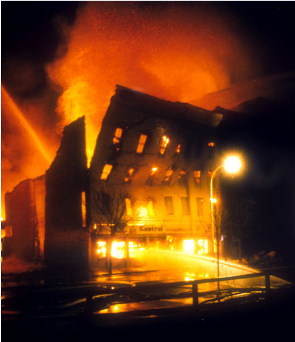
Figure 3. Fire Causing Collapse of a URM Building
