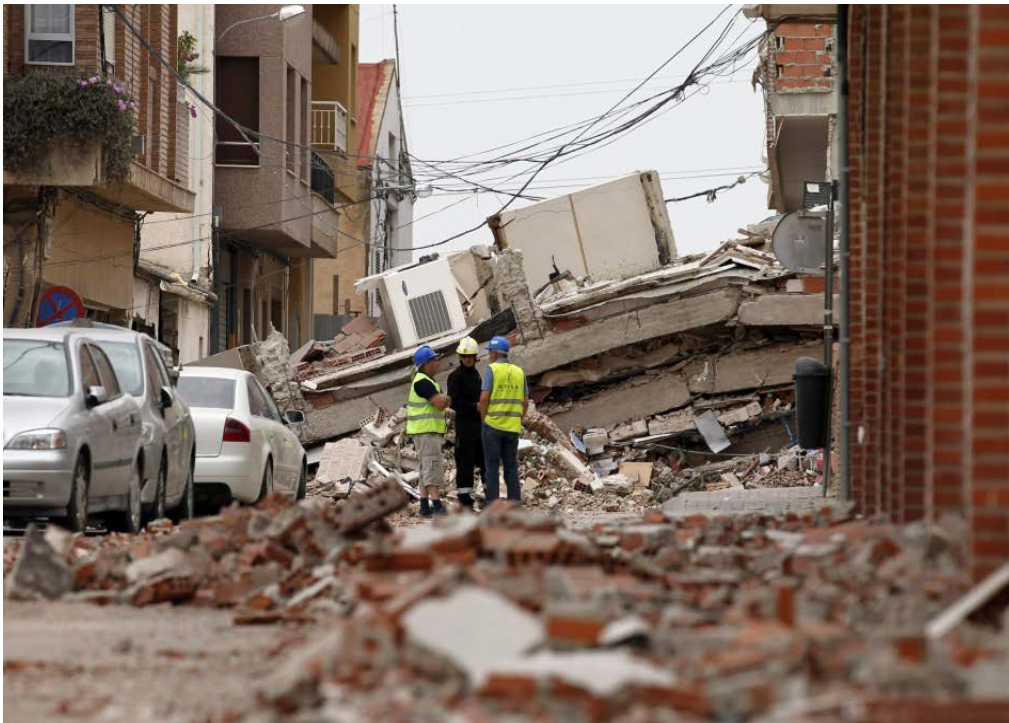
Figure 1. Damage to URM buildings Following the 2011 Lorca Earthquake in Spain
