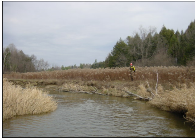
Figure 6.15. Tree Revetments in M10.
