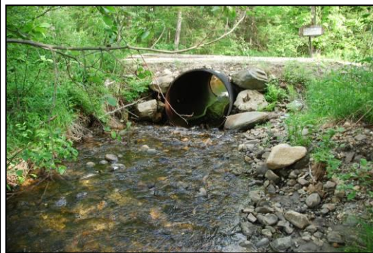
Figure 7. Perched and undersized culverts along reach M10S1.02 (left) and M09S1.02 (below).
