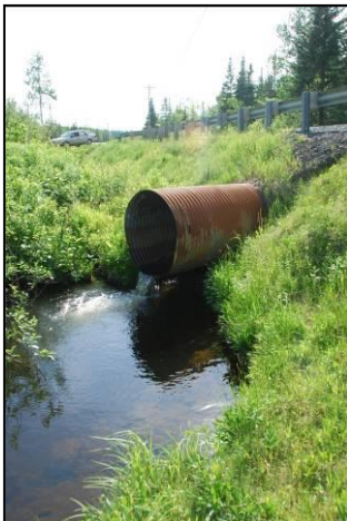
Figure 7. Perched and undersized culverts along reach M10S1.02 (left) and M09S1.02 (below).
