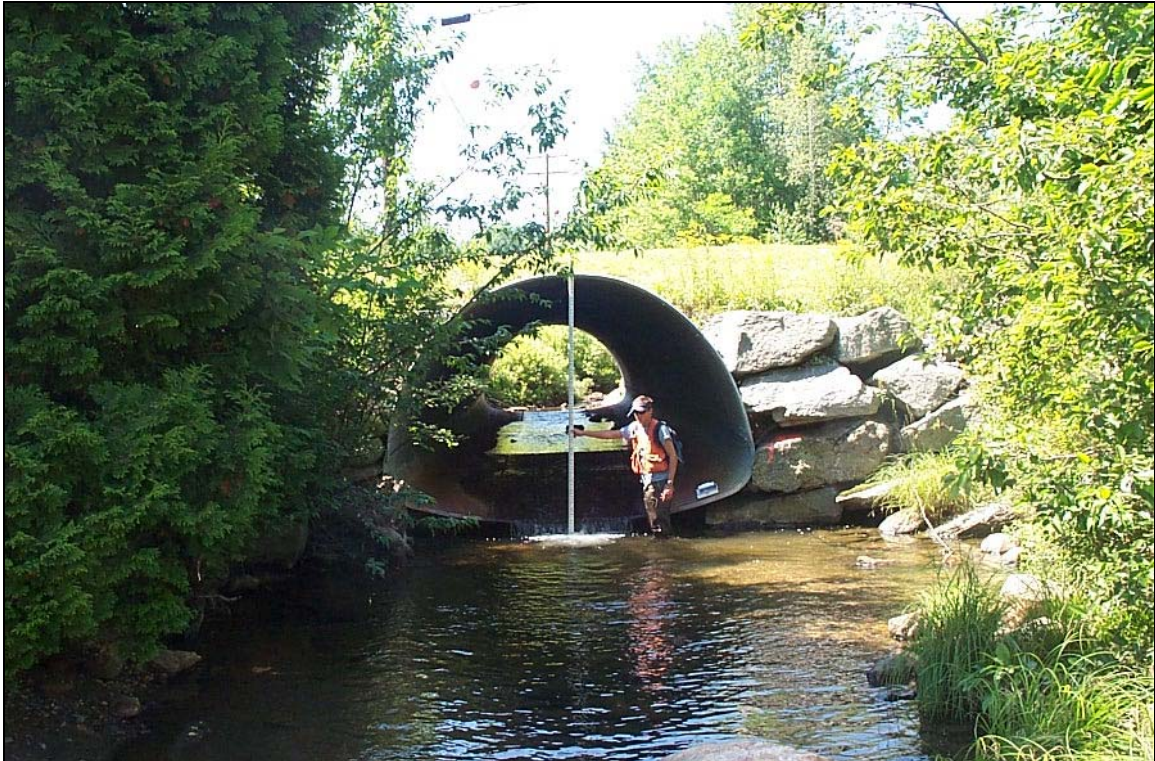
Figure 34: Undersized culverts disrupt the sediment transport capacity of the stream and may lead to both upstream and downstream destabilization. Improperly sized structures, such as this one on T2.13-A, can interfere with sediment transport and create scour below the structure.
