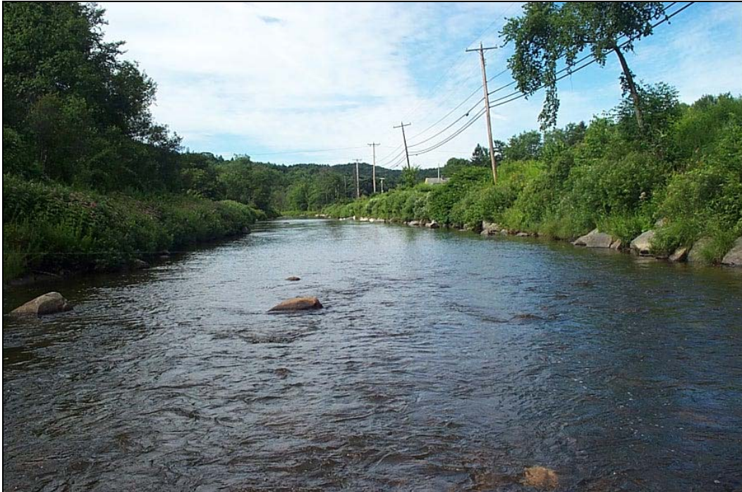
Figure 16: Segment T2.04-B has been extensively straightened and confined by Route 100. It is now a “B” type channel with a plane bed form.
