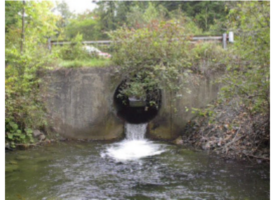
Figure 4. The invert of the culvert outlet. Outlet of structure #56 is free fall.
