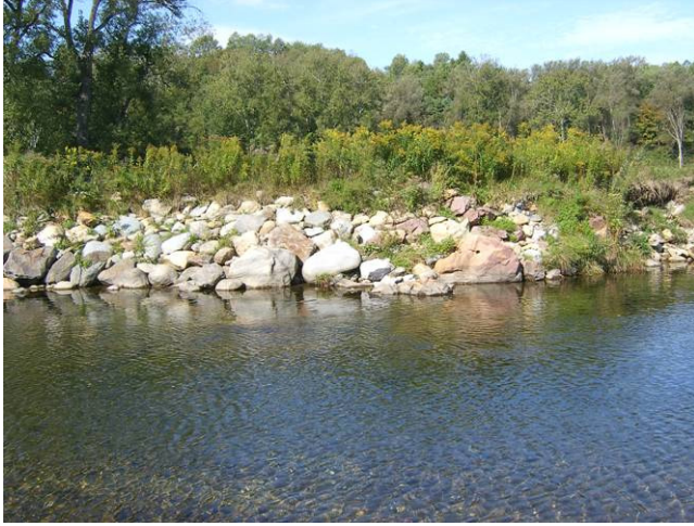
Figure 3: Rock revetment and lack of buffer at Reach M06's left bank
