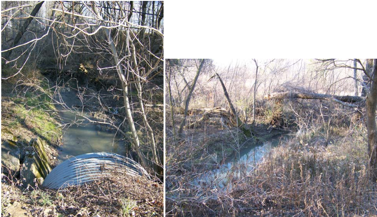
View of a culvert and bank erosion (L) and the stream channel (R).
