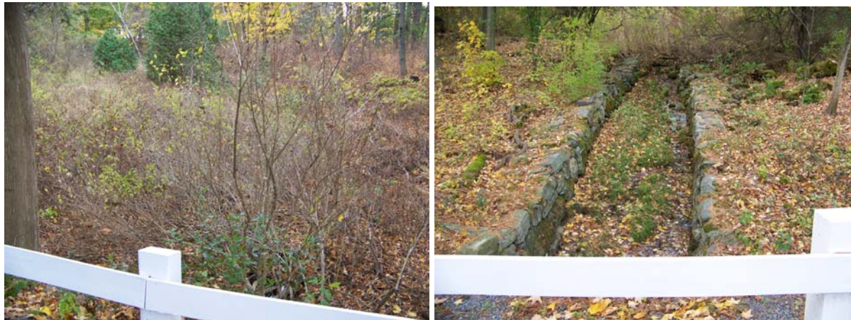
Riparian area (L) and old riprap/channelization (R).
