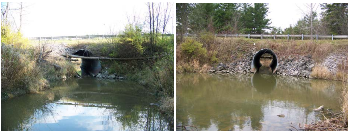
Upstream (L) and downstream (R) views of the southern (upstream) culvert. Note the woody debris upstream and scour downstream.
