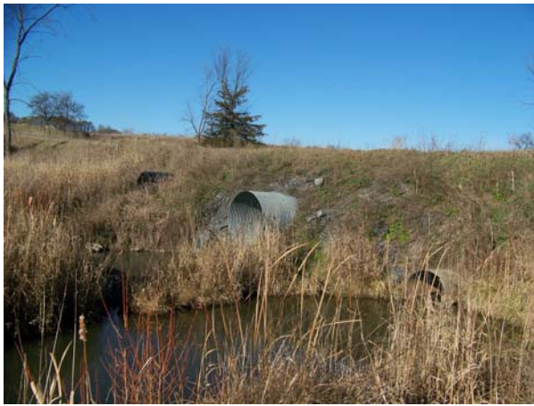
Culverts with overflow pipes (L) and beaver activity (R).
