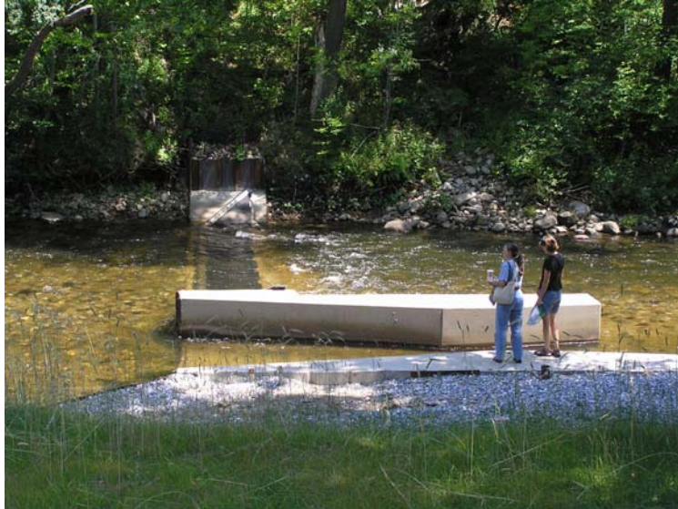
Figure 12. Water withdrawal intake structure for Okemo Mountain snow making located on the Black River (reach M34) in Ludlow. 29 May 2006.
