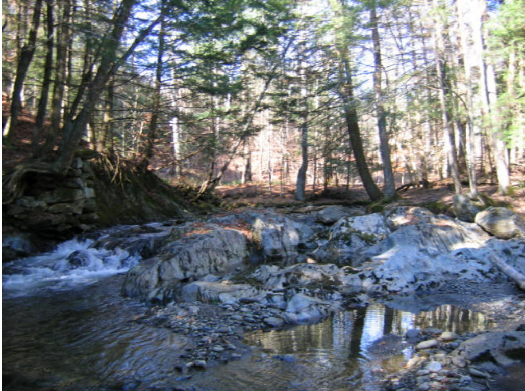
Figure 15. Bedrock grade control in middle of reach R13S3.03
