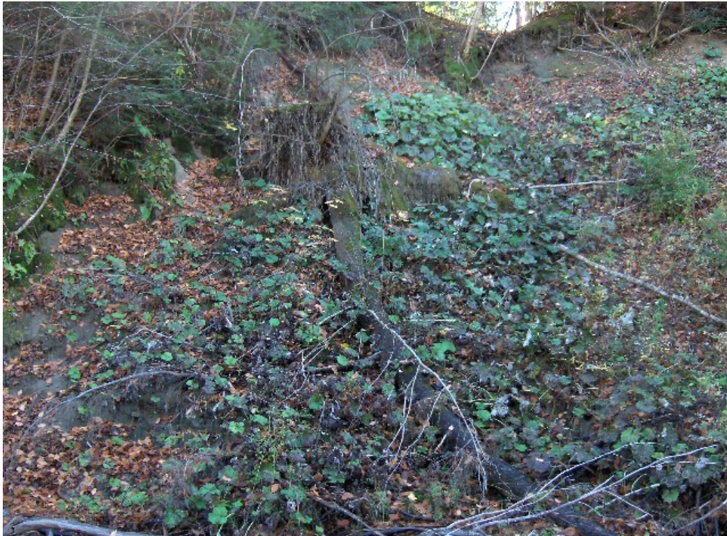
Figure 6. Mass Failure in segment R13S03.01-B
