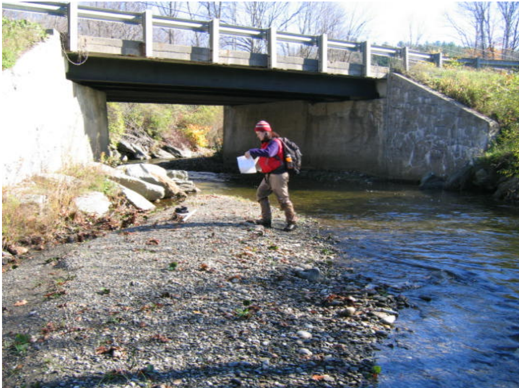
Figure 11. Deposition below Route 15 Bridge in R13S3.01-C
