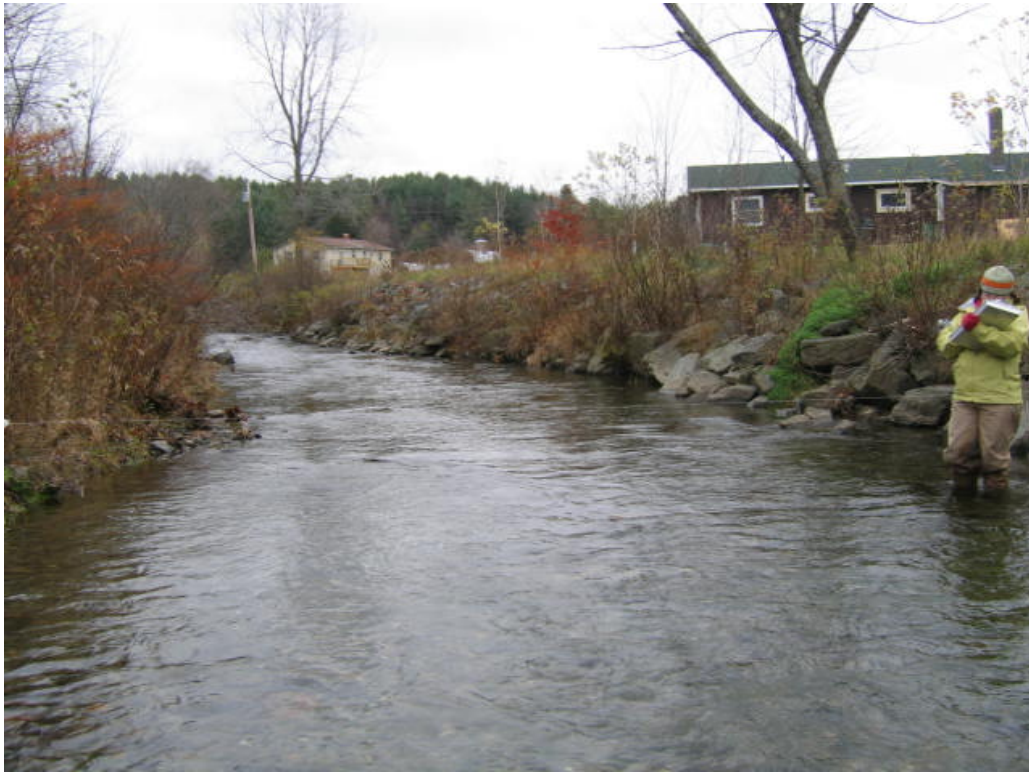
Figure 9. Rock riprap along southern bank in R13S3.01-C
