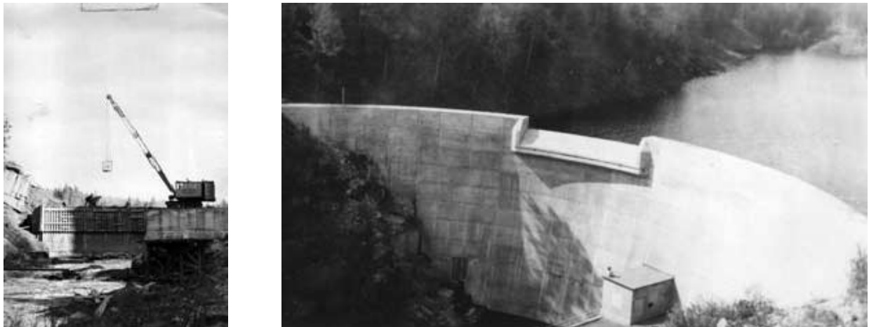
Figure 9: Historic images of the Green River Dam, from A Brief History of the Green River Project and the area covered by it , Willard K. Sanders, 1951.
