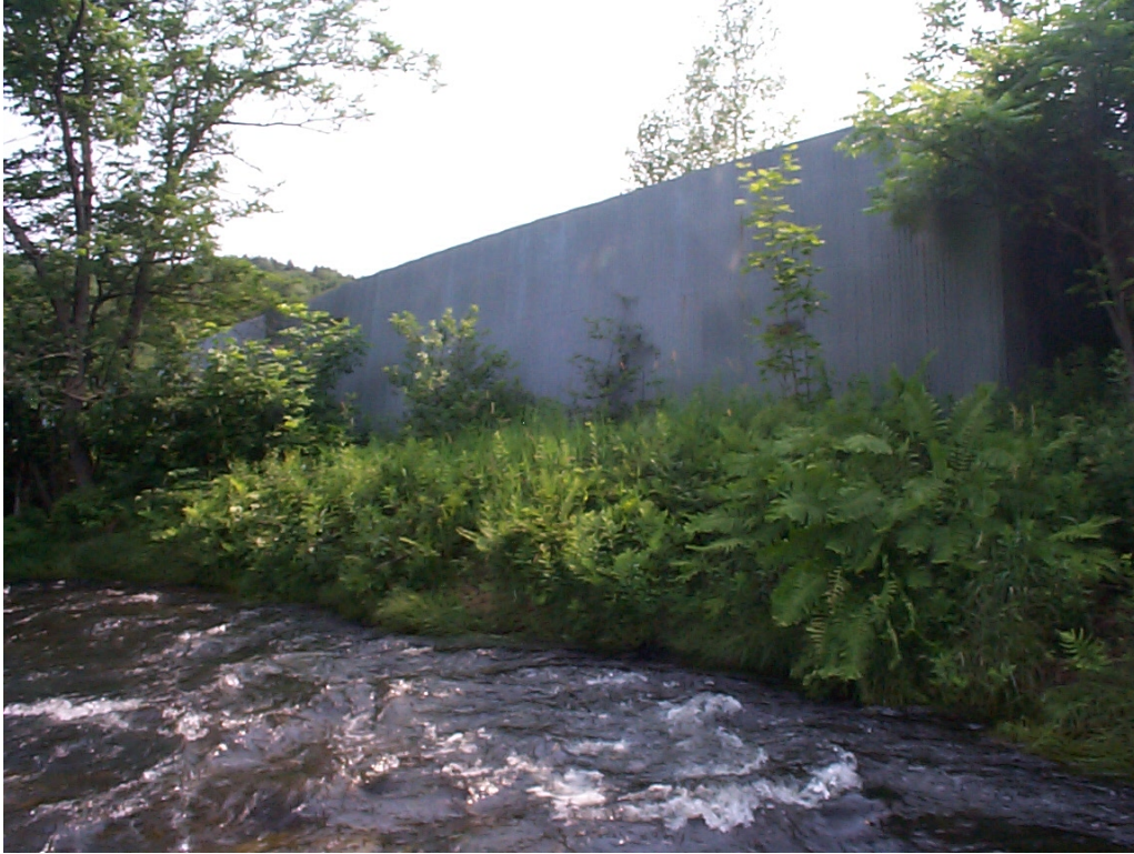
Figure 11: Reach M01 – Floodplain encroachment from junk yard behind the large fence.
