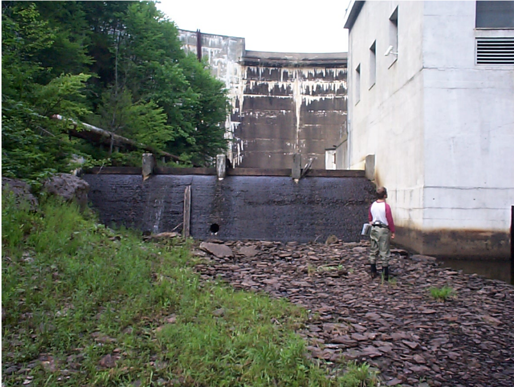
Figure 2: Reach M12 – Dam at Green River Reservoir.
