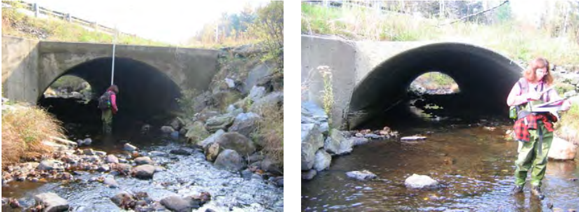
Figure 12. Inlet (top left) and outlet (top right) of Garfield Road arch
