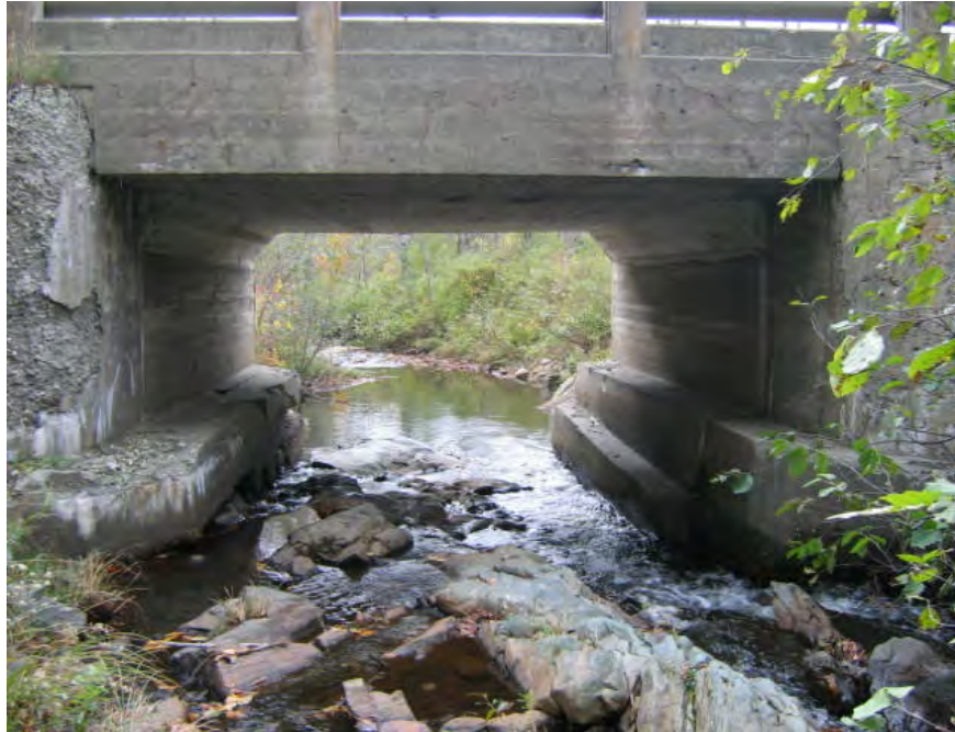
Figure 7. Bedrock grade control at Route 15 Crossing
