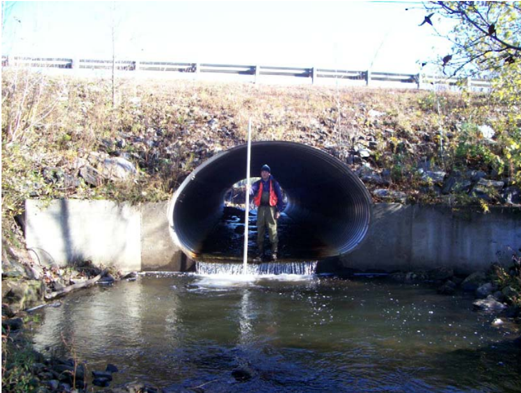
Figure 10. Culvert at Centerville Road in reach R15.07-B was flagged as “No Aquatic Organism Passage” using the Vermont Culvert Aquatic Organism Passage Screening Tool (Milone and MacBroom, Inc, 2008)
