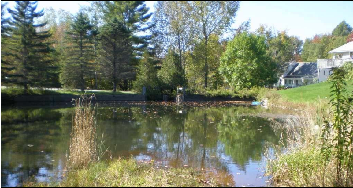
Figure 11. Segment M10-B is an on-stream pond controlled by a small concrete dam.
