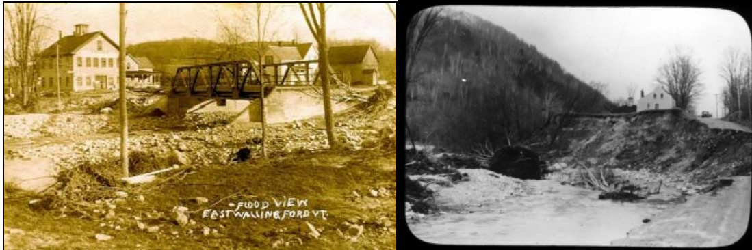
Figure 3: These images of the nearby Mill River show damage from the 1927 flood. Left image is looking towards the intersection of Route 104 and Route 155 in East Wallingford. Right image is of route 103 washout in Cuttingsville. (Similar damage was likely inflicted on land around the Cold River).
