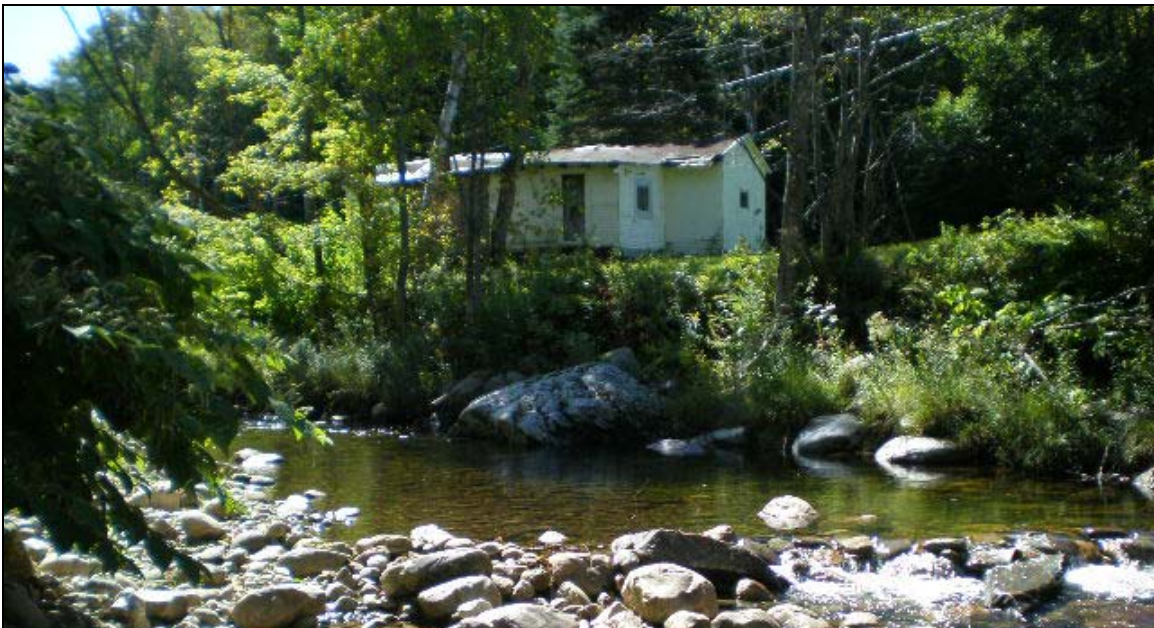
Figure 21. M06 flows along Cold River Road and has been impacted by channel management activities meant to protect public and private property that was built in the river corridor.
