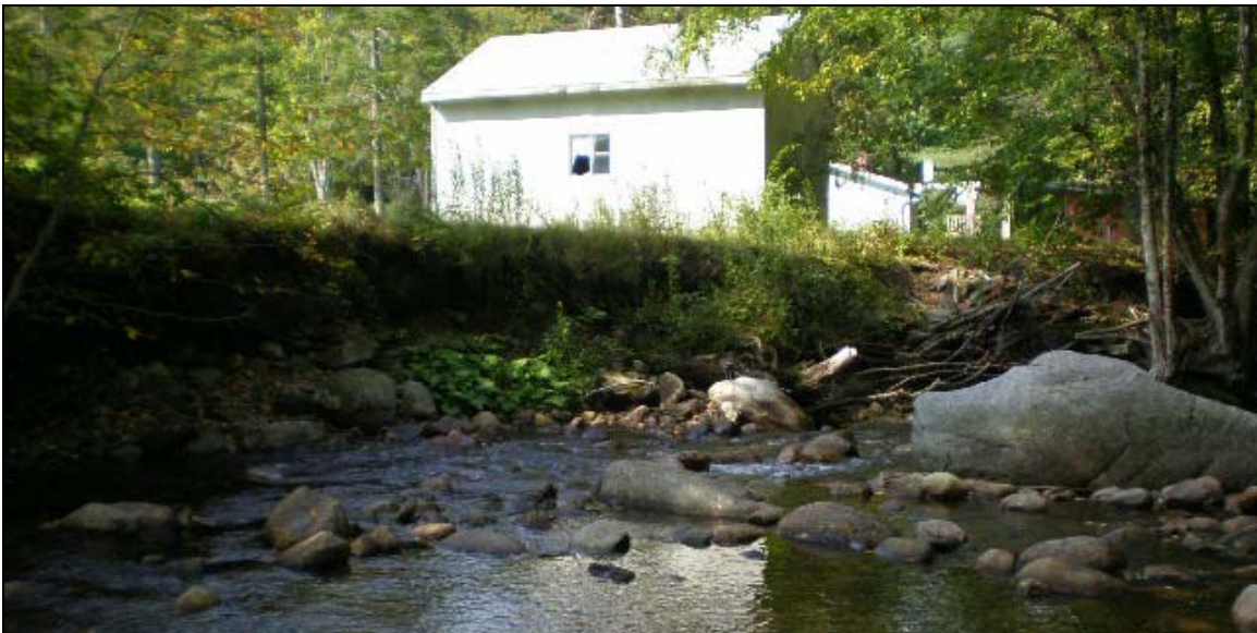
Figure 19. M07-A has a significant degree of floodplain encroachment as well as channel management evidence such as berming, straightening, and bank armoring.
