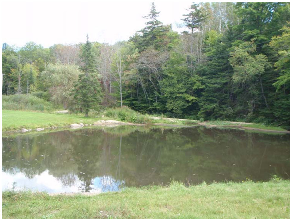
Figure 4.8 Impoundment behind dam in Segment M10-B
