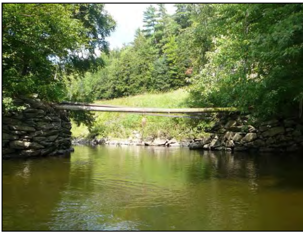
Figure 39. Old abutment serving as a channel constriction
