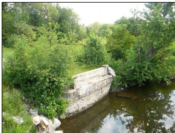
Figure 19. Old bridge abutment
