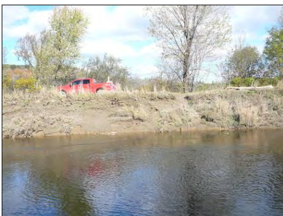
Figure 10. Erosion and poor buffers at the cross section
