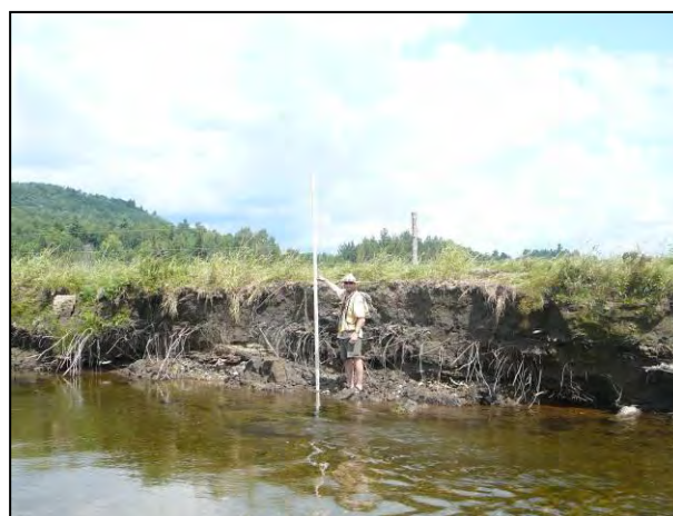
Figure 38. Erosion of outside meander bend and poor buffer condition
