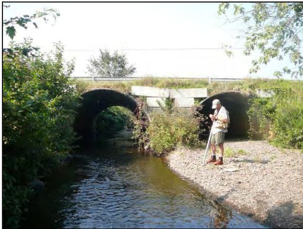
Figure 25. Double Culvert associated with Loop Road crossing
