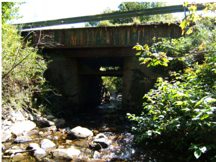
Figure ff. Morse Road Bridge, Segment B
