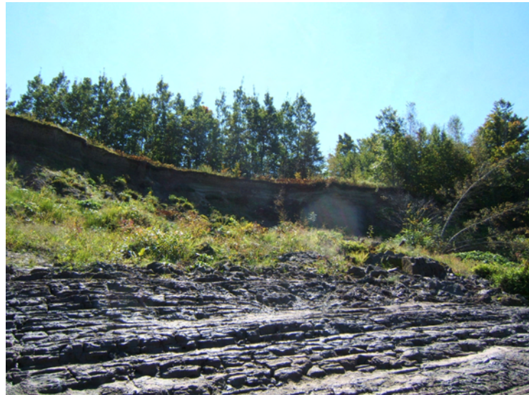
Figure h. Mass Failure in Main Branch Reach R16
