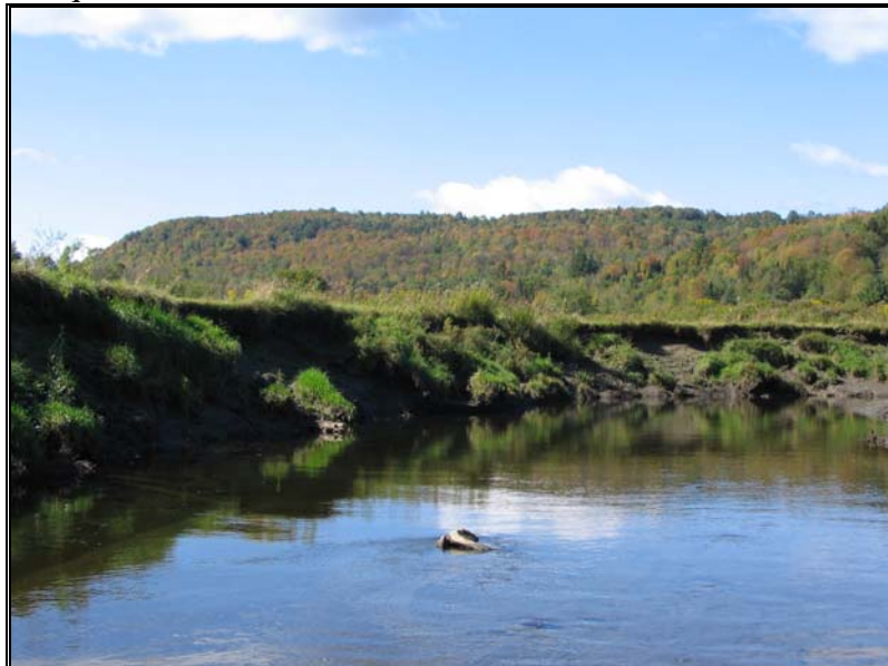
Signs of Degradation on Reach 31 Winooski River; Photo taken by TJC
