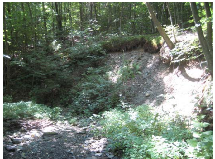
Photo 4: Dry section and erosion on sharp, outside bend upstream of a culvert. Again, note deposition upstream of bend.
