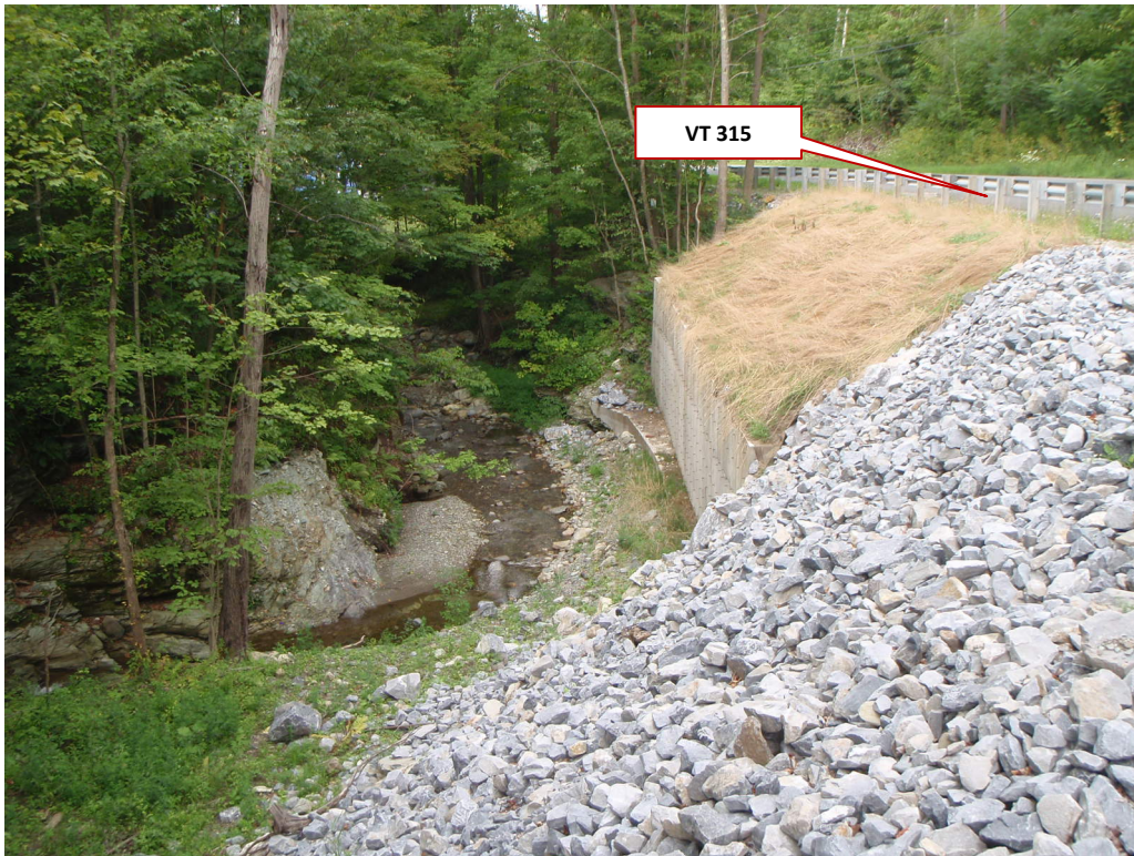
Figure 4.7 Encroachment of VT315 on Mill Brook corridor. Example of using a vertical wall to minimize road encroachment for road-river compatibility. Reach M01T1.03.
