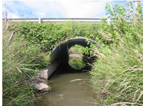
Figure 7. Culvert beneath Route 2A
