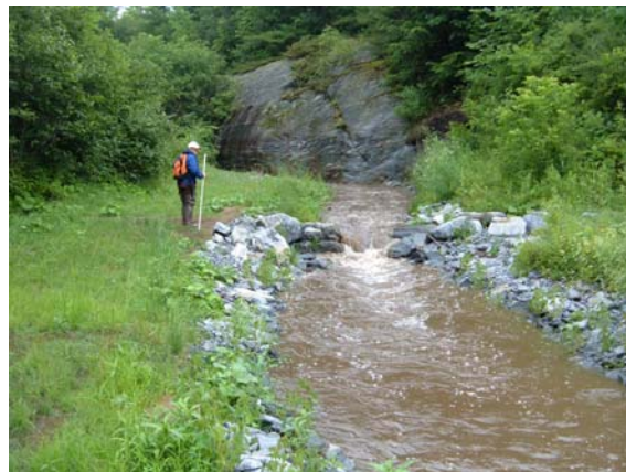
Figure 13. Channel restoration site in upper T1.02
