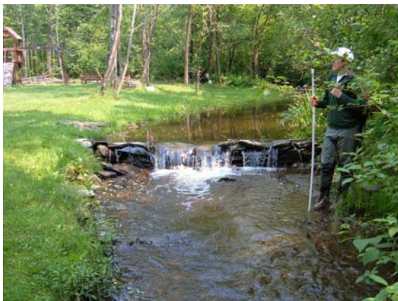
Figure 16. Rock weir in lower Segment T1.04-B
