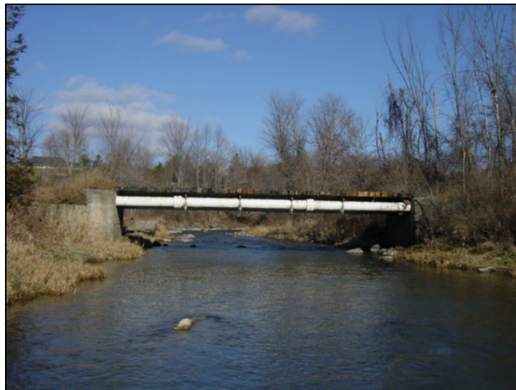
Farm access bridge in M06.
