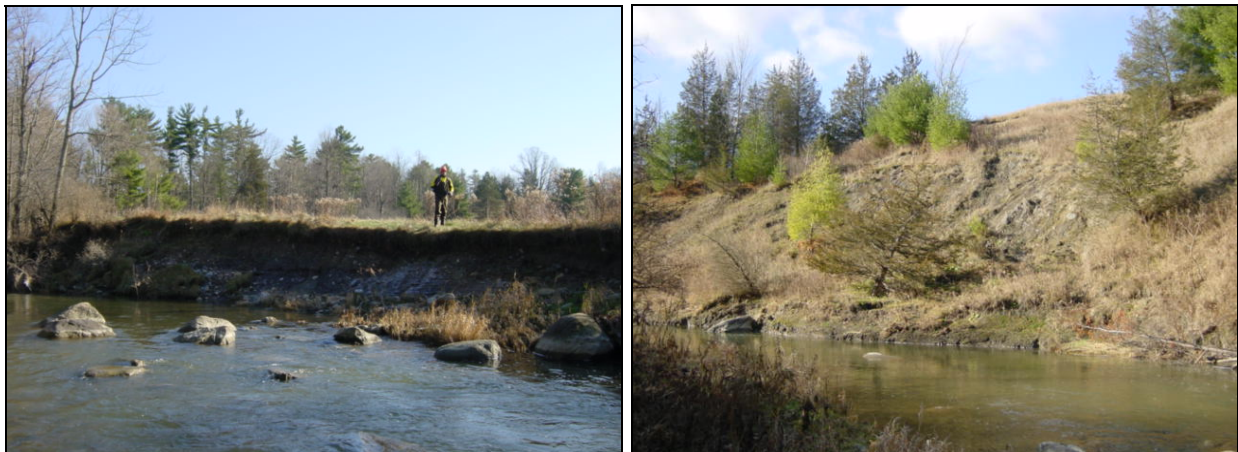
Bank erosion on an outside bend, contributing sediment (L) and one of many mass failures in M06 (R).
