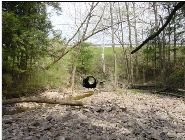
Bostwick Rd crossing in T1.05A with large sediment deposits and channel widening upstream.
