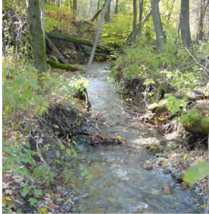
Figure 8b. Extreme effects of constricting the channel and blocking flow of sediment has led to property damage with aggradation upstream and erosion downstream.
