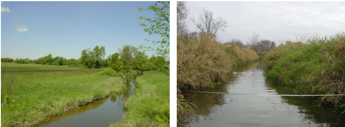
Figure 3. Straightening and lack of woody riparian vegetation affected RGA and RHA condition in Hinesburg.
