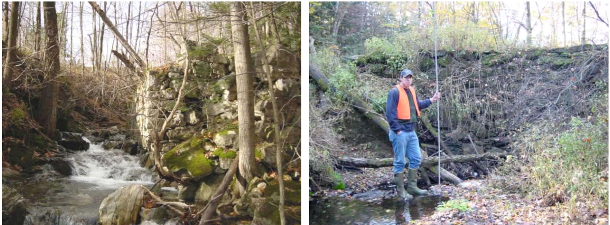
Figure 6. Mill footing on Beecher Hill Brook T5.01C (left) and mill dam on Patrick Brook T4.04 (right).
