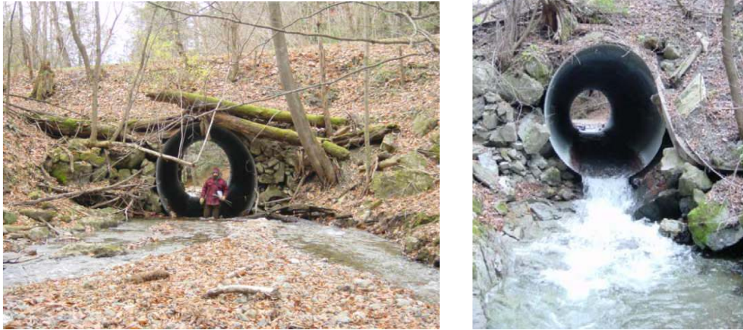
Figure 7. Beecher Hill Brook (T5.01B) culvert. Note aggradation forming bars and splitting flow upstream. Some erosion was noted downstream, although the downstream end falls onto ledge and boulders.
