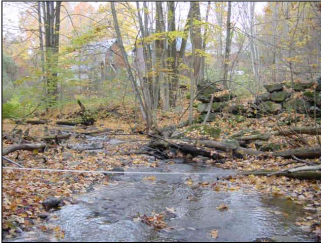
Reach view with old abutment.
