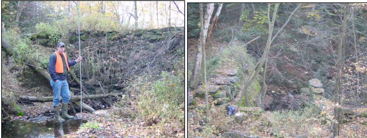
Old mill dam upstream and downstream photos.
