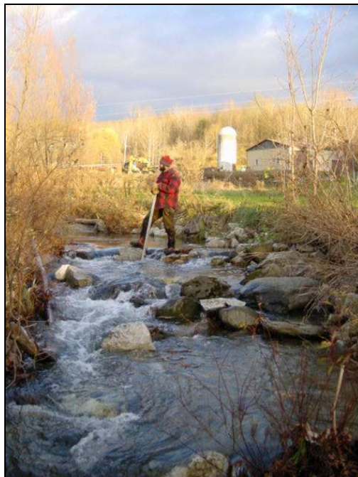
Headcut downstream of Beecher Hill Rd.
