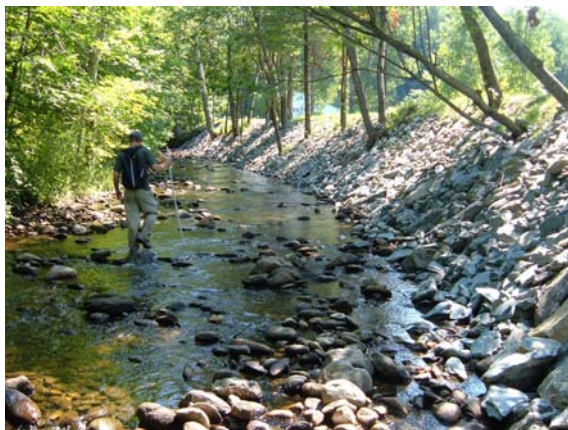
Figure 14. Armoring along reach M13-A
