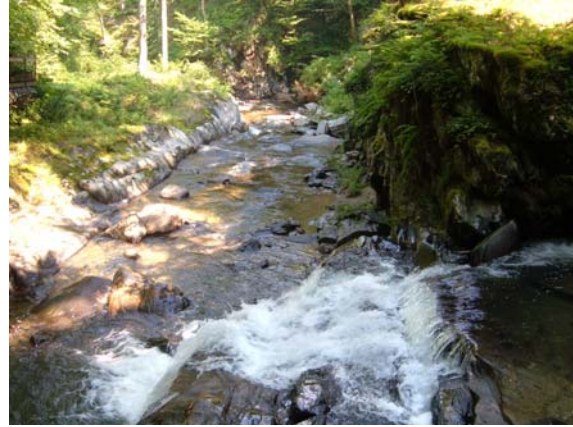
Figure 4. Grade control mid-reach in M04
