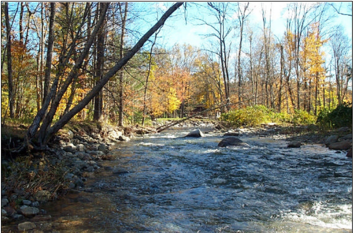
Figure 14. Reach M3.05 is undergoing active planform adjustment. A flood chute cuts across the inside of this meander (right bank) as the river migrates left causing trees to fall into the river.
