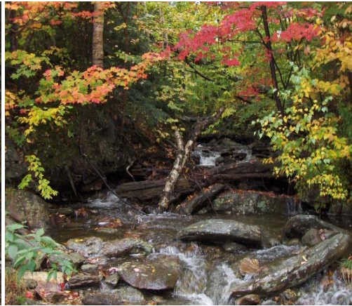
Figure 7.34. Active head cut and bank erosion in segment M08.S1.03 of Big Spruce Brook
