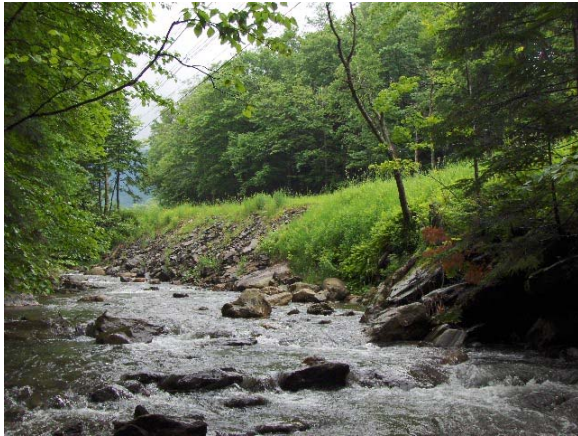
Figure 7.14. Straightening and armoring of M09-A along Route 108 causing lack of riparian buffer and decreased floodplain access
