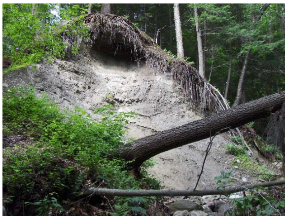
Figure 7.18. Mass failure in segment M07.T5.01.S1.01-A
