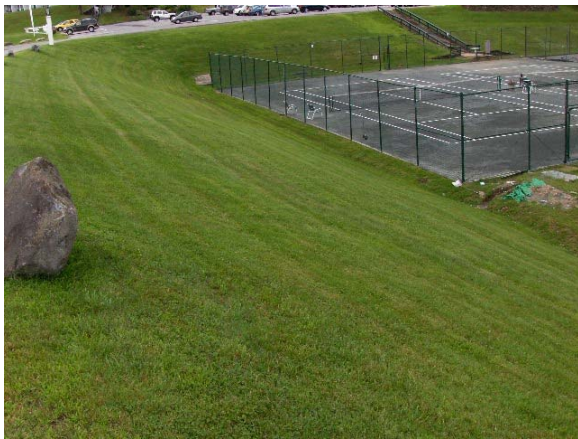
Figure 7.22. Location of underground culvert in M07.T5.01.S1.01-C
