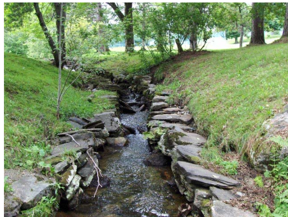
Figure 7.23. Channel straightening and armoring in M07.T5.01.S1.01-C
