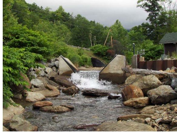
Figure 7.13. Downstream view of weir in M08-C
