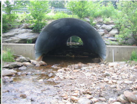
Figure 7.36. Significant sediment deposition above undersized culvert on Longtrail tributary
