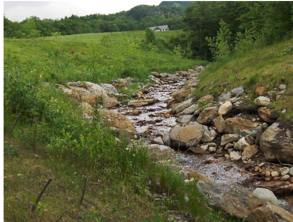
Figure 7.32. Reconstructed channel in segment M08.SI.03-A
