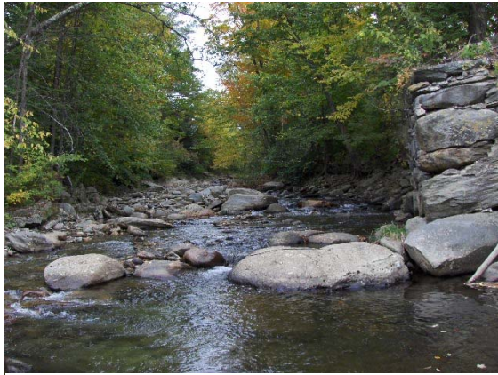
Figure 7.1. Straightened channel and old abutment in Segment M07-A
