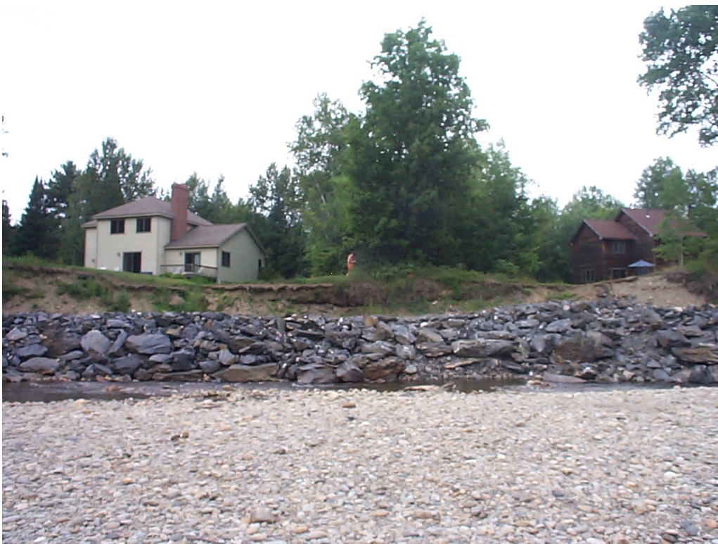
Figure 9. Rip-rapped erosion threatening residential structures on the West Branch
