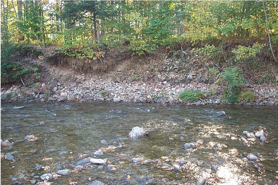
Figure 14. Erosion on Reach 4
