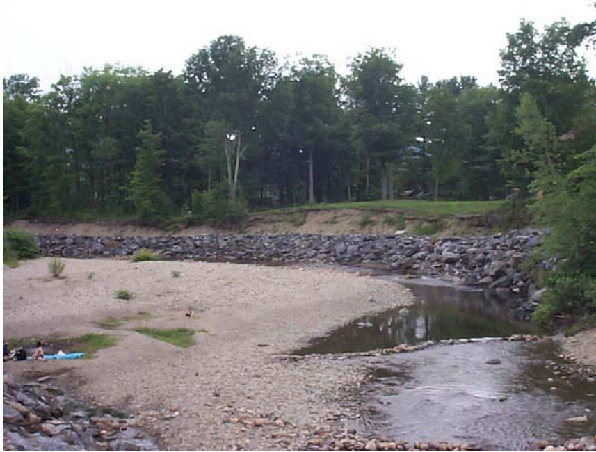
Figure 12. Sediment upstream of Luce Hill Bridge
