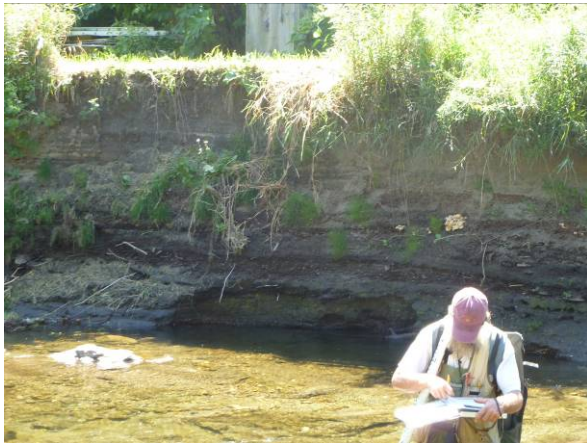
Figure 13. Legacy sediments behind the old dam at Ben’s Mill show a distinct pattern of banding indicating cyclic deposition over the years the dam was in place; a heavy sediment discharge and subsequent erosion have occurred since the dam breached (around 1990).
