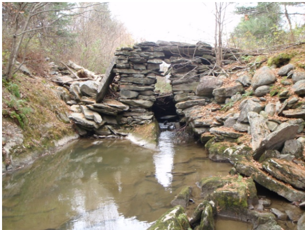
Figure 4.21 Looking upstream at the channel constriction
