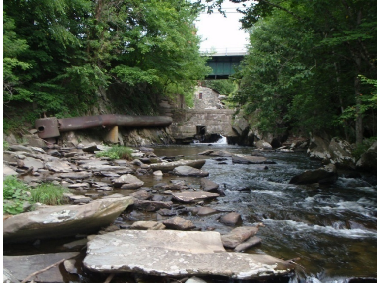
Figure 4.38 Dam and penstock downstream of Rt. 15 crossing
