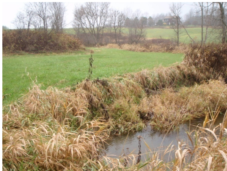
Figure 4.28 Bank slumping and buffer width < 25 feet on the left bank
