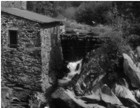
Figure 4.39 The dam at the Old Red Mill c. 1964 (UVM, 2009)
