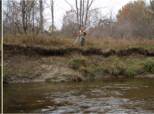
Figure 4.14 Severe erosion along left (west) bank in upper M06
