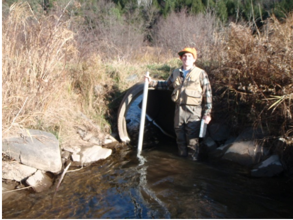
Figure 4.34 Culvert inlet looking downstream
