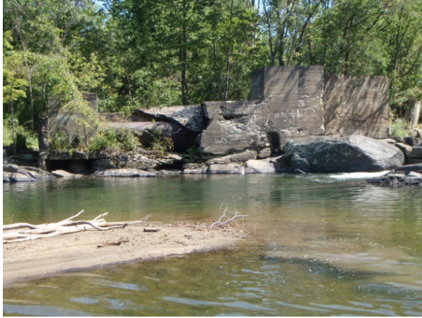
Figure 4.9 Remnants of dam/hydro-electric facility
