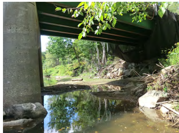
Figure 5.2. The stream channel is split by a pier under the Higley Hill Road bridge. Sediment is filling one side and blocking flow.
