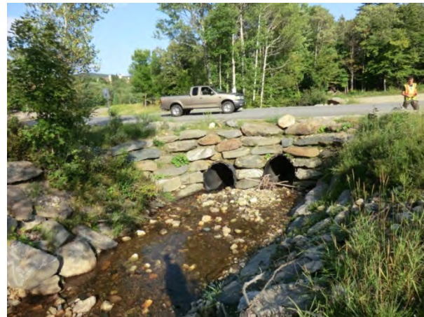
Figure 5.4. The Handle Road culvert is perched. Figure 5.5. North Access Rd. culverts are causing deposition.
