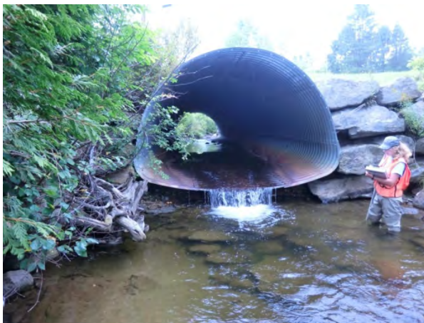
Figure 5.4. The Handle Road culvert is perched. Figure 5.5. North Access Rd. culverts are causing deposition.
