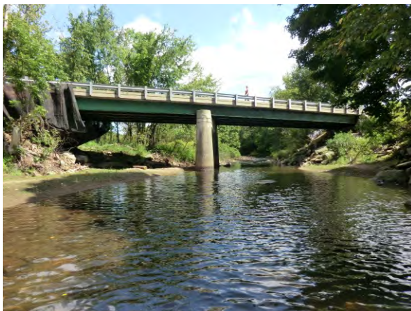
Figure 5.2. The stream channel is split by a pier under the Higley Hill Road bridge. Sediment is filling one side and blocking flow.
