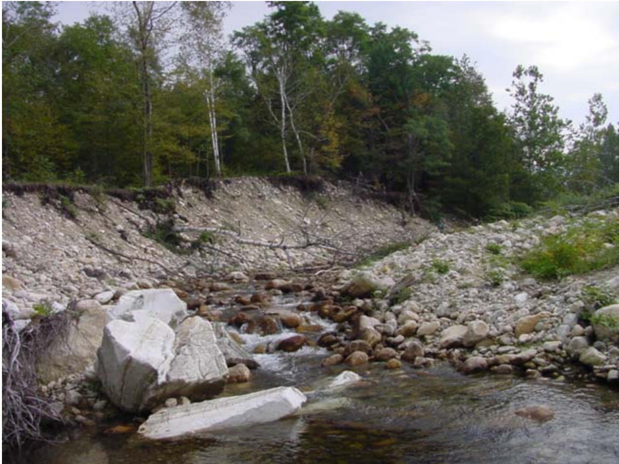
Figure 3-5: Bank Erosion Upstream of Park Street.
