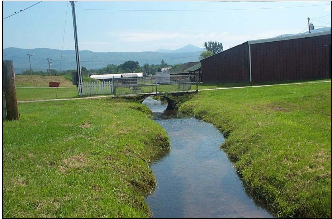
Figure 23: Typical cross section through segment M22-SI.01-SI.01-B. Channel straightening, floodplain encroachments, undersized structures, and no riparian vegetation typify this reach.
