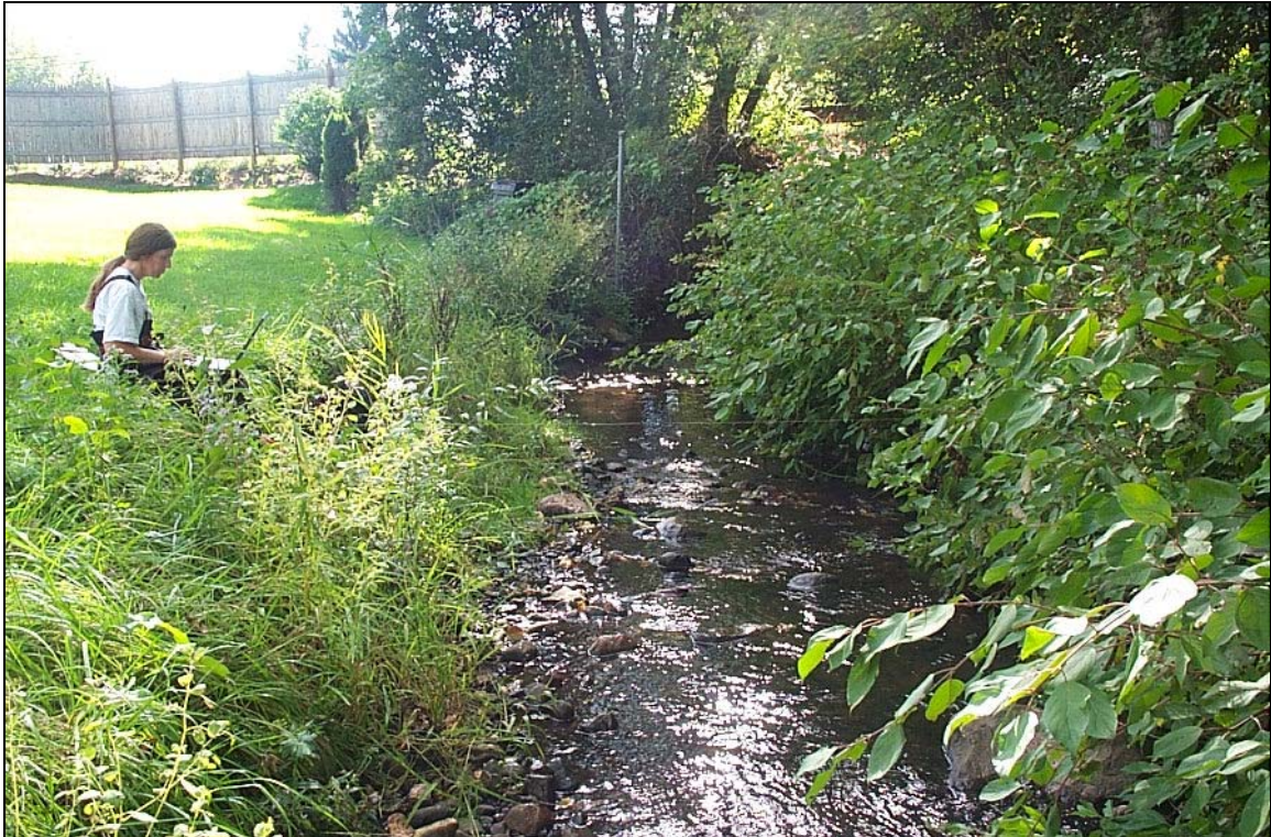
Figure 17: Segment M22-SI.05 is an E4 riffle-pool system that has been altered by development in the floodplain and historic channel straightening. Streamside vegetation (as along the right bank of the photograph) has been disturbed along much of the reach.
