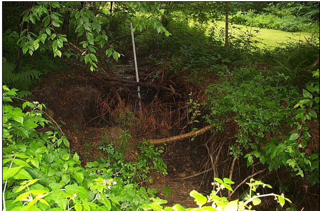
Figure 19: An active head cut is seen in this photograph of segment M22-SI.08-A. Downstream of the white survey rod the stream has incised approximately three feet exposing tree roots and the streambanks to fresh erosion.
