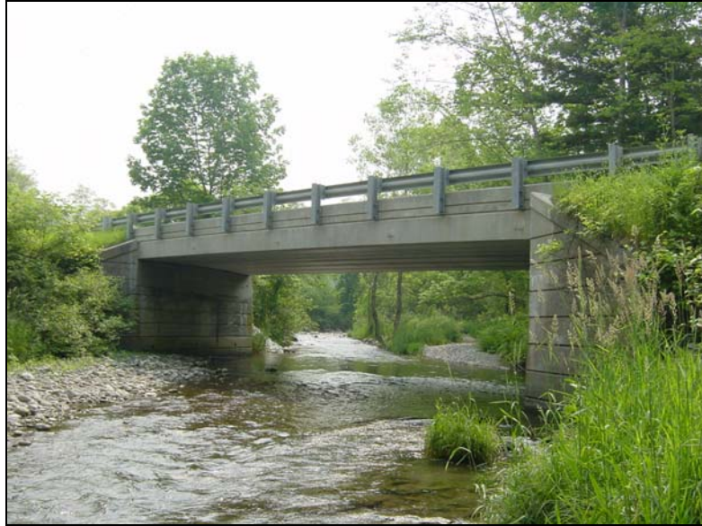
Figure 10. Sediment deposited upstream of this bridge on M14A. Photo view is looking upstream through the bridge.
