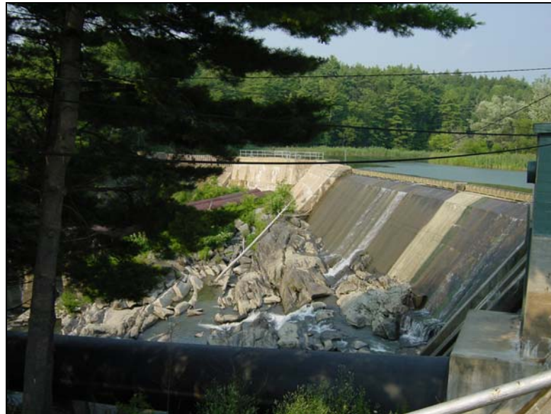
Figure 4. Carver Falls Dam between Reaches M04 and M05.
