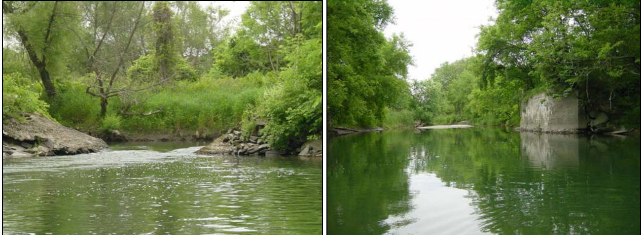
Left photo is abutment highlighted in Figure 16. Right photo is upstream of Route 22A.
