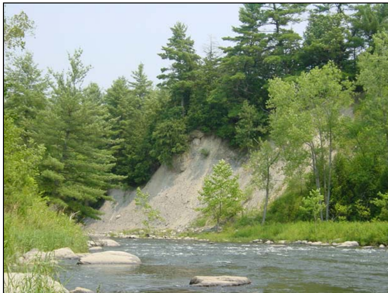
Figure 23. One of several mass failures in reach M05 resulting in reduced habitat and geomorphic condition.
