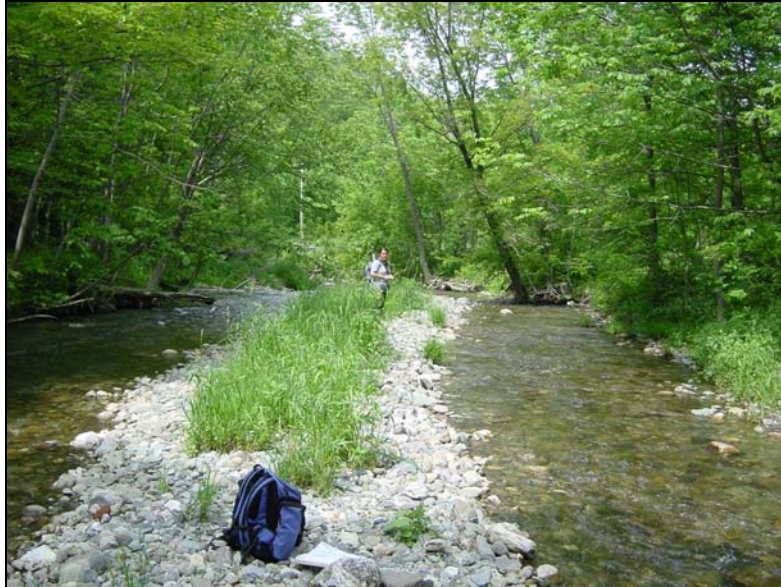
Figure 12. Sediment deposition upstream of a bridge channel constriction on M14A.
