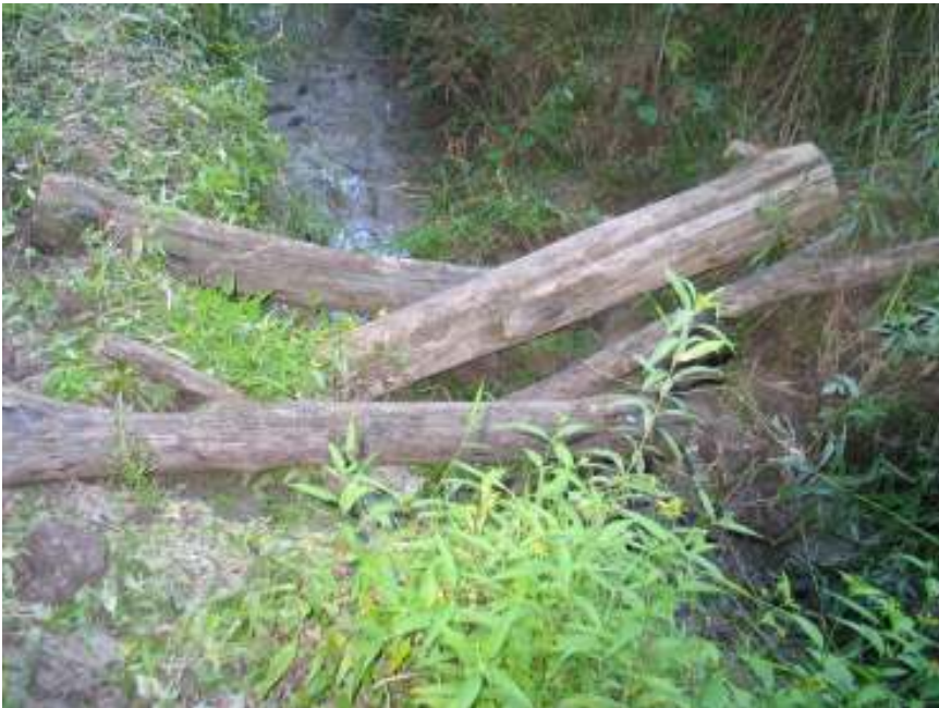
Figure 6: Channel-spanning woody debris placement to create a new debris jam and trap sediment.
