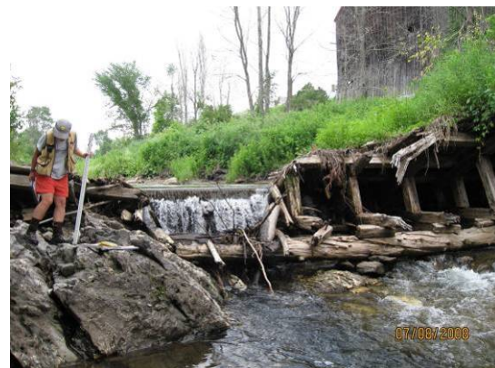
Figure 20. Aggradation upstream (left) of a partially breached dam (right) on the Tabor Branch indicates likely ongoing “sediment starving” downstream.
