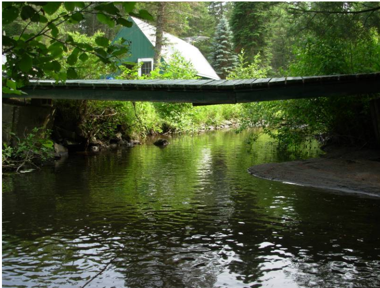
Figure 69. Development encroachment in segment T1.09C; bank toe stabilization placed on both banks; bridge is a channel constriction with some deposition noted upstream
