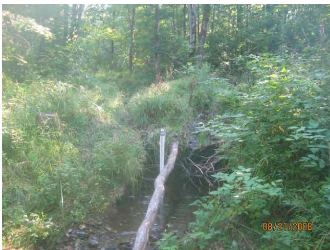
Figure 76. This headcut is moving up a road in the Branon sugarbush on segment T2S1.04D. Several headcuts like these are impacting the roads as well as posing the potential for extending the stream network, increasing flows in the stream while eliminating access to valuable floodplains.
