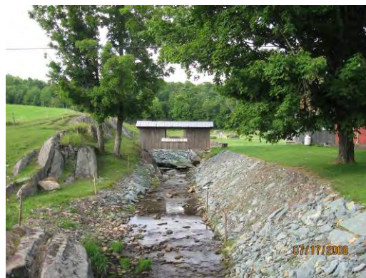
Figure 88: Reach T4.01, segment A has been straightened most of its length. The upper portion of the segment has created new floodplain (left), while the downstream end has been completely armored to prohibit lateral movement.
