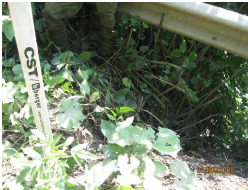
Figure 31. Bank failures triggered by stormwater inputs that carry runoff from road ditches to a perched culvert above a steep valley wall in segment M14A have repeatedly cut back the road edge (left) and triggered mass failures on the valley wall below (right). The area was heavily ripped in early 2009. Japanese knotweed in the picture at left was one of the few incidences of invasive plants evident in reaches assessed in 2008, and might be limited from further spread by a rapid response.
