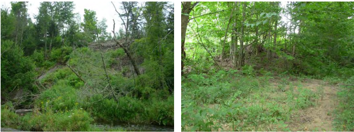
Figure 47: Bogue Branch, reach T2.01, segment C. A large mass failure is found below Bogue Rd. on the left bank valley wall in mid-segment (left). Summer downpours contributed to sediment inputs to the stream from a farm road off the right bank (right).
