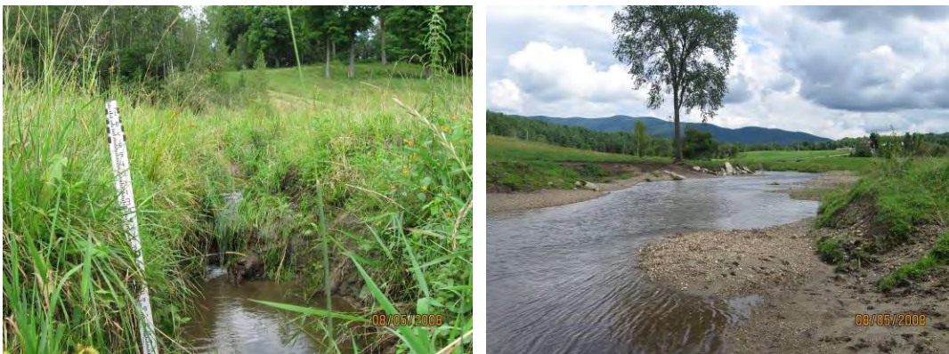
Figure 50. Nickpoint in a field ditch entering Bogue Branch T2.02C (left) may have been related to recent intense storms rather than the limited amount of stream incision noted in the segment. Gravel removal in the upstream portion of the segment (right) was part of the basis of straightening noted for the segment.
