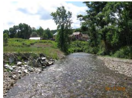
Figure 54. FEMA helped fund riprapping of the left bank in segment T2.04A beneath the Lopes' home and barns at Witchcat garlic farm, which has been augmented by windrowing and berm construction upstream.
