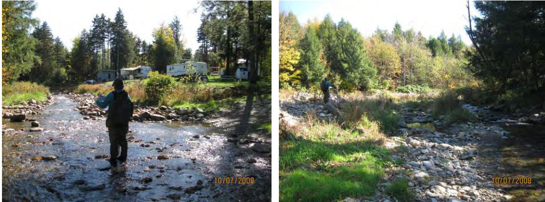
Figure 18. Sediment windrowing (left) and small-scale stockpiling (right) in reach M13.
