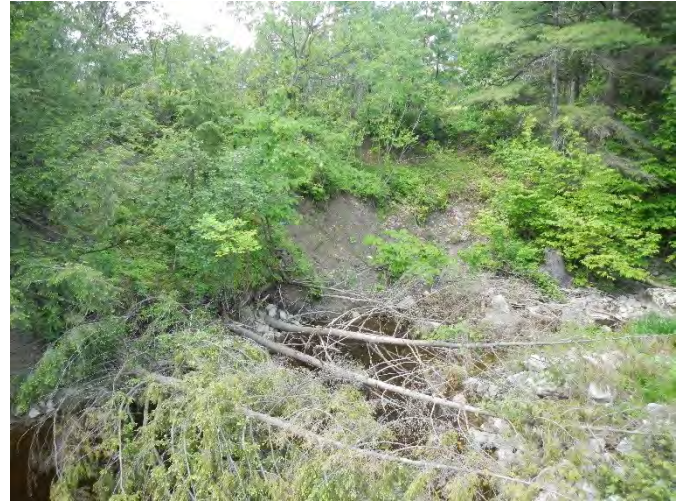
Figure 19: Small mass failure on QT3.01.
