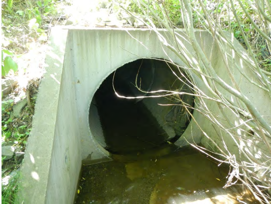
Figure 11: Road culvert on QT3S1.01.
