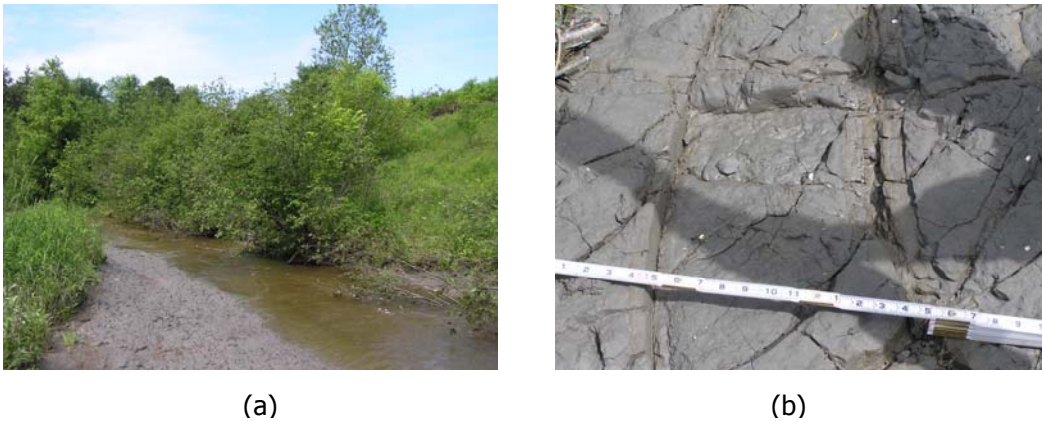
Figure 18. M06. A 120-foot channel-spanning exposure of varved clays serves as a local vertical grade control for the channel. (a) view downstream (b) closeup view of varved clays exposed above 6/13/2006 water level on the inside of the meander bend.
