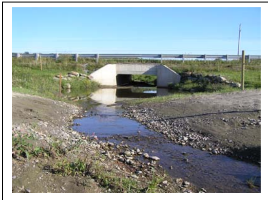
Figure 15. T3.3S1.01 – Section B. NRCS-engineered cattle crossing approximately 75 feet downstream of Chester A. Arthur Road crossing – installed August 2005.
