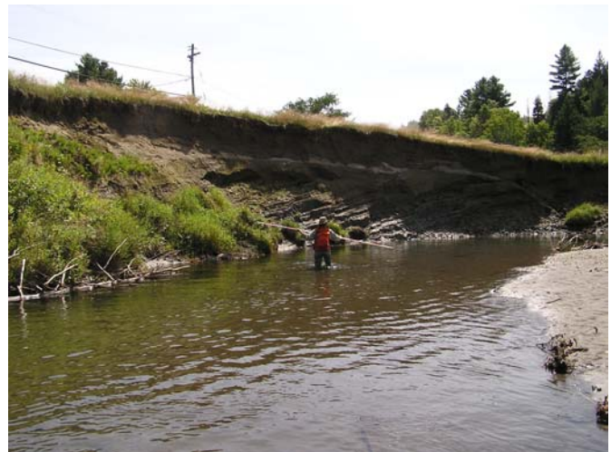
Figure 14: Reach T201 showing mass failure and lateral migration
