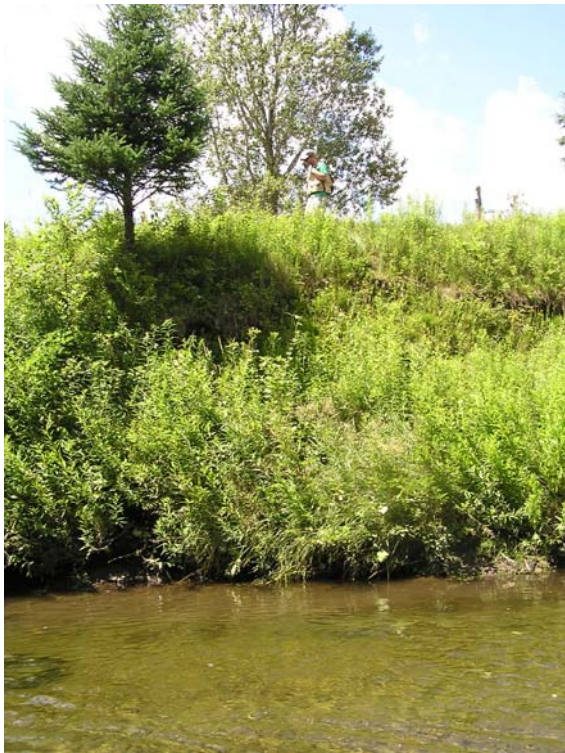
Figure 18: Photo showing right bank of Miller's Run Reach T202 with slumping banks. The gravel operation is along the corridor on this side of the river
